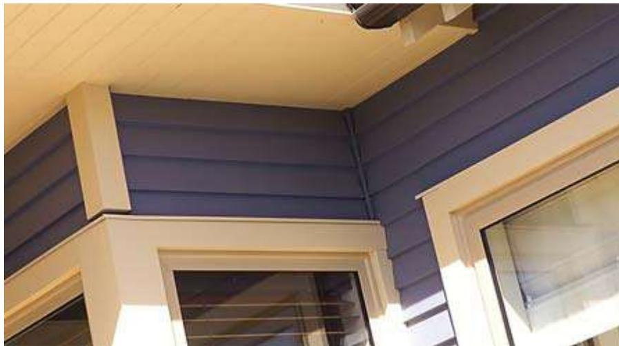
**Eaves.** Properly designed eaves can provide the correct amount of shading and protection for windows and external doors as well as being sympathetic to the coastal aesthetic.
