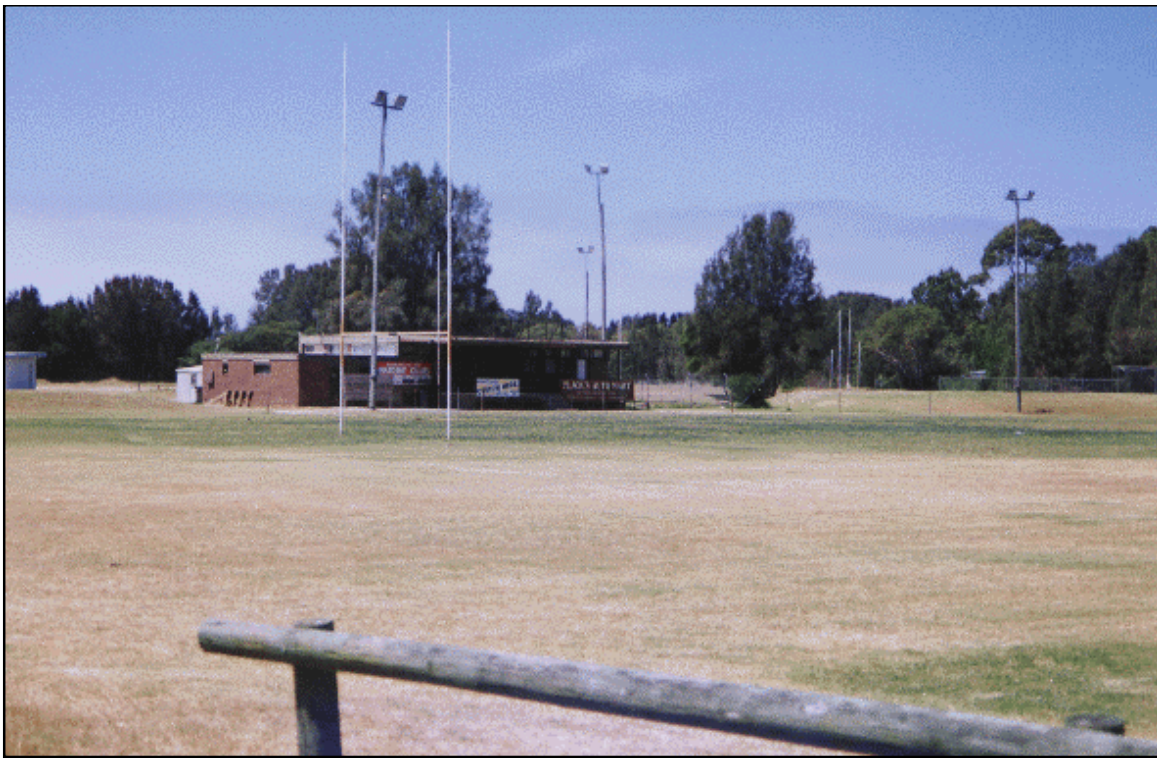
Pictured is the Rugby Union oval in the foreground. The proposed new multiuse amenities building and kiosk will be located to the left of the existing Rugby Union Clubhouse building and will be shared by Australian Rules, Soccer and Rugby Union ovals.
