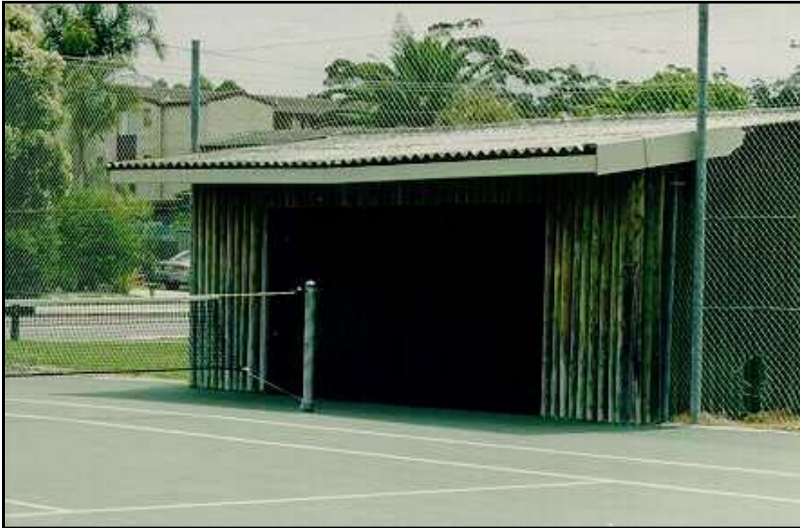
Tennis courts shelter
