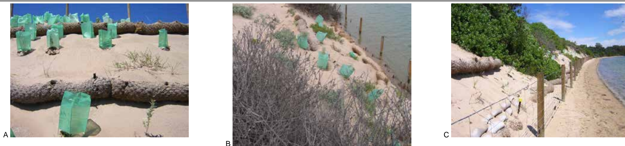
Figure 71: Coir log terrace, original fence and revegetation at Tomakin Spit
