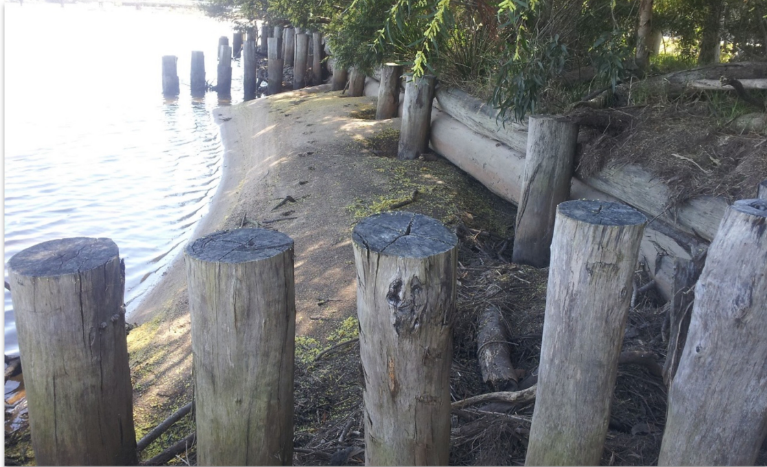
Figure 6.5 Example of timber groynes in the Murrumbidgee River
