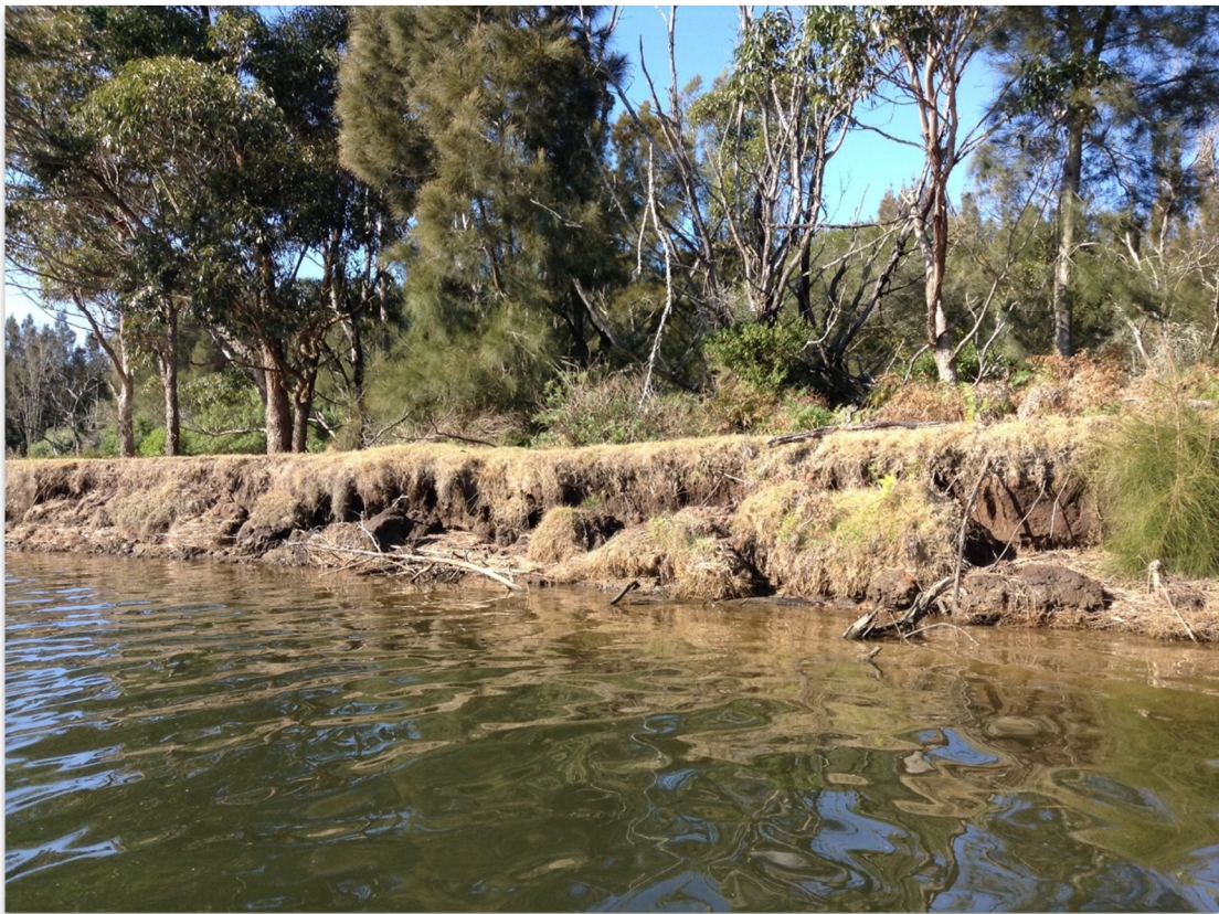
Figure 3.8 Bank erosion on north-west side of Cambathin Island
