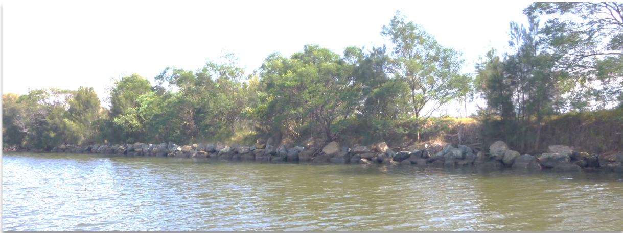
Figure 6.4 Example of a rock revetment in the main channel of the Tuross River
