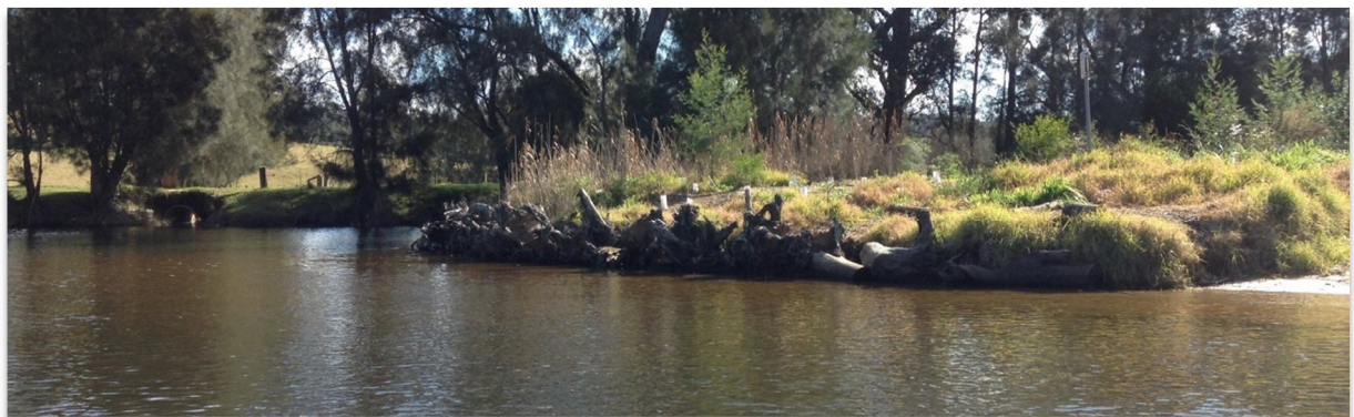
Figure 6.6 Example of a woody debris in the Tuross to protect an exposed section of bank
