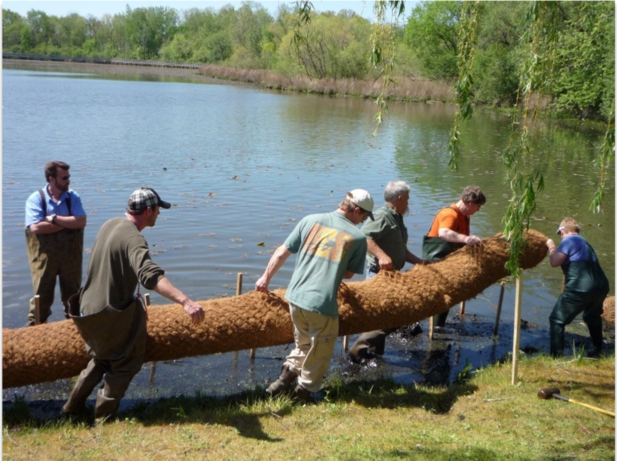
Figure 6.2 Example of coir log installation ( http://www.hrwc.org/2010/05/building-a-natural-alternative-to-breakwalls/ )
