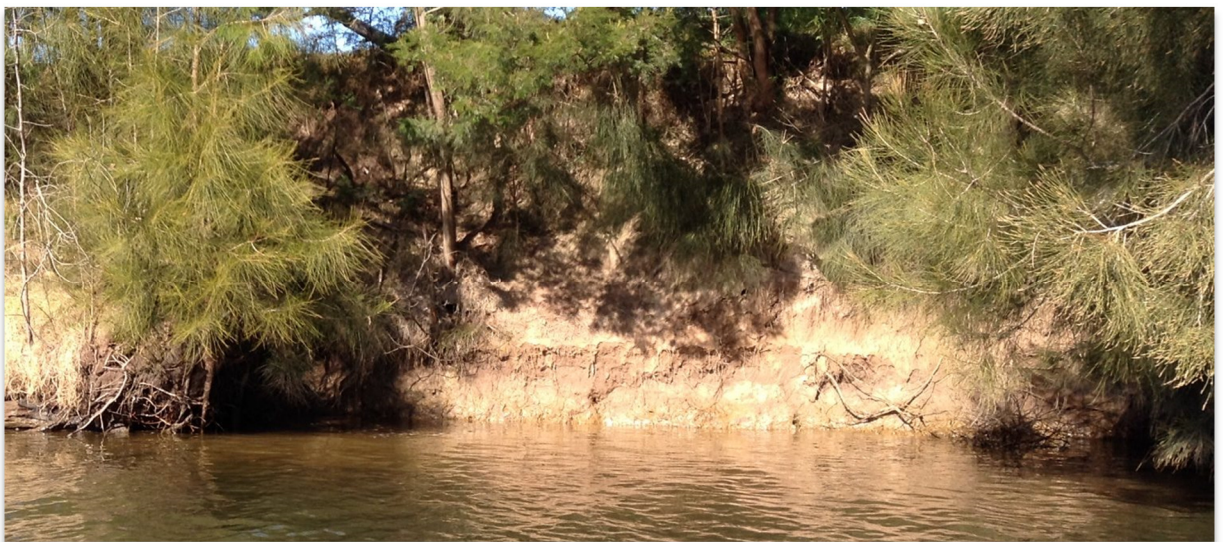
Figure 2.4 Example of recent bank failure as a result of flows being directed at this bank
