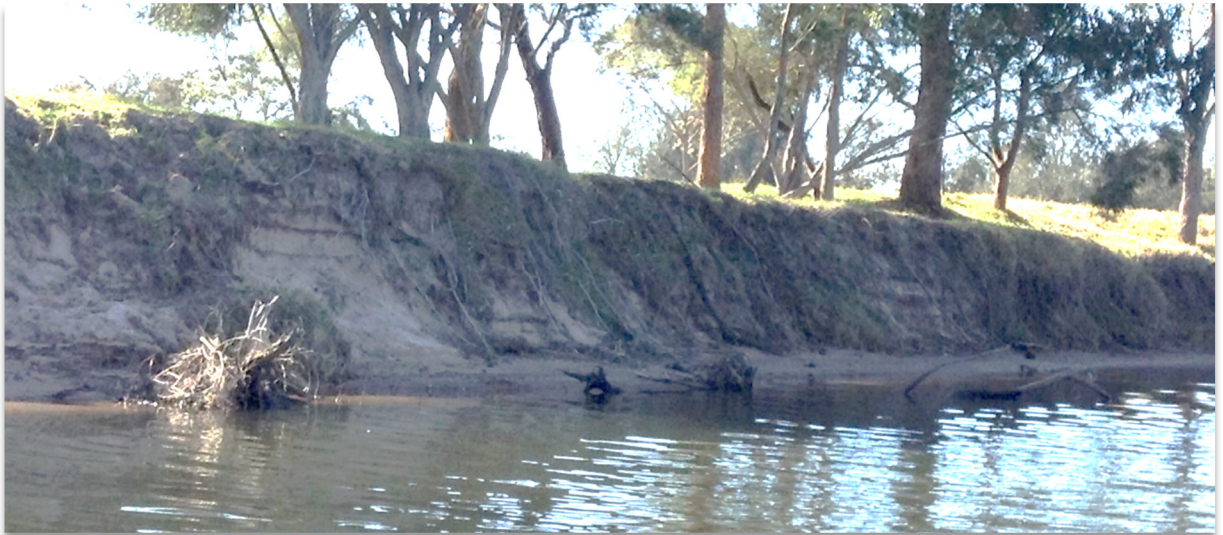
Figure 2.3 Example of an exposed sandy sub vertical bank with active erosion
