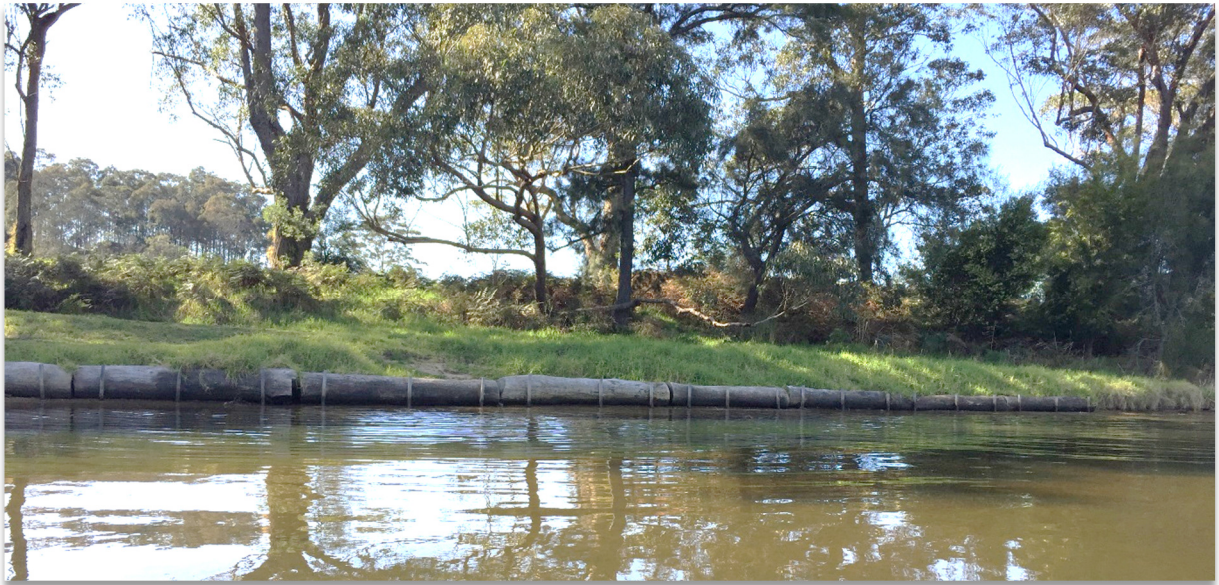
Figure 6.3 Example of a log structure at Snake Flat
