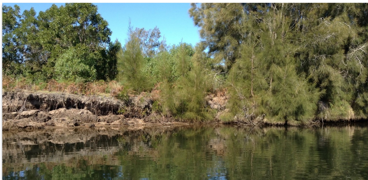
Figure 4.1 Cambathin Island, note clump of casuarinas adjacent to section of failing bank. This may a suitable location to start rock and reduce the risk of outflanking.
