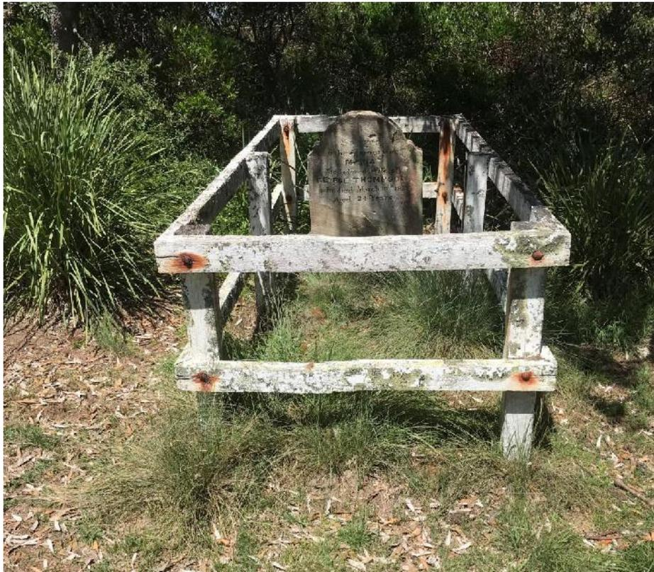
Photo showing active rust in the bolts and some timber splitting around the bolts. PG
