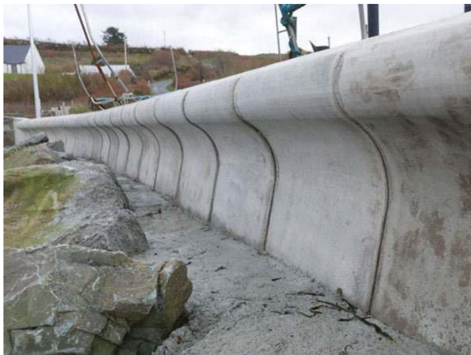
Figure 7 Example of a concrete wall return barrier
