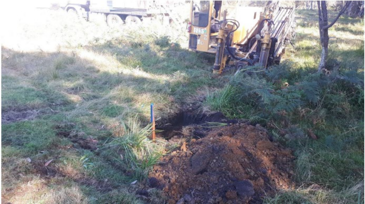
Photo 4: HDD equipment installing street main
