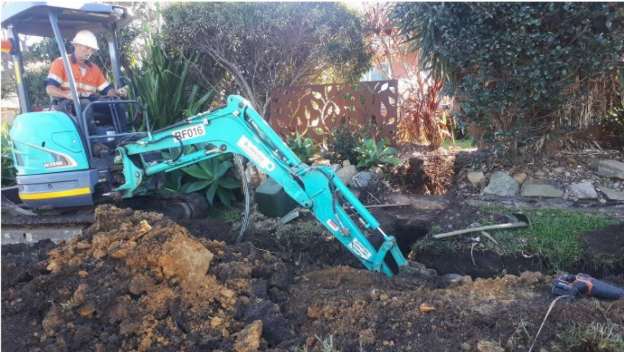
Photo 2: Excavation for pressure sewer lateral and boundary kit
