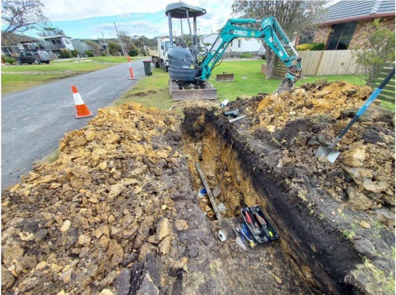
Photo 3 Excavation for isolation valve and wye connection
