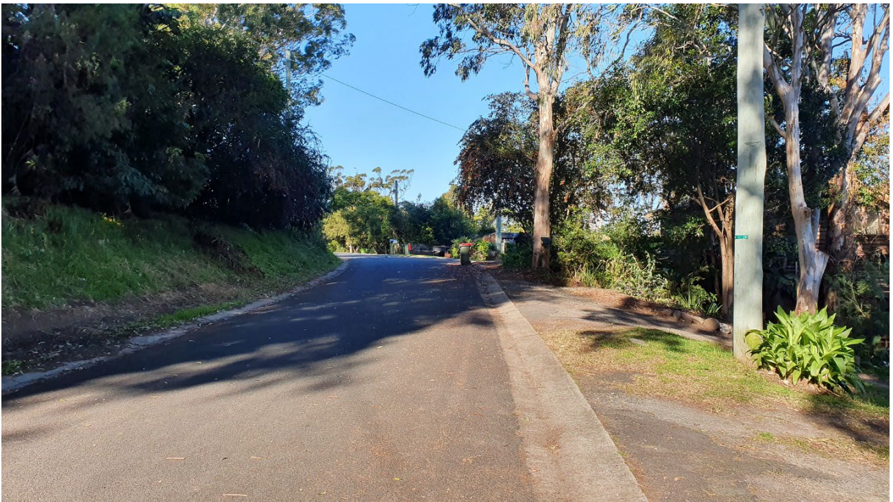
Photo 11: Turner Lane looking south
