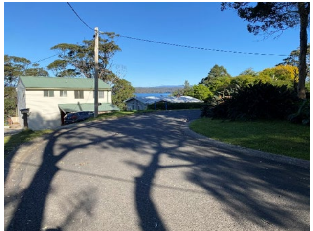
Photo 45: View west along Flower Circuit Drive showing electrical services, residences built into east-west slope and view towards Wallaga Lake
