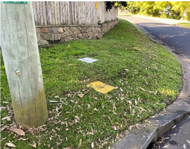
Photo 44: View west showing installation of services along Flower Circuit Drive
