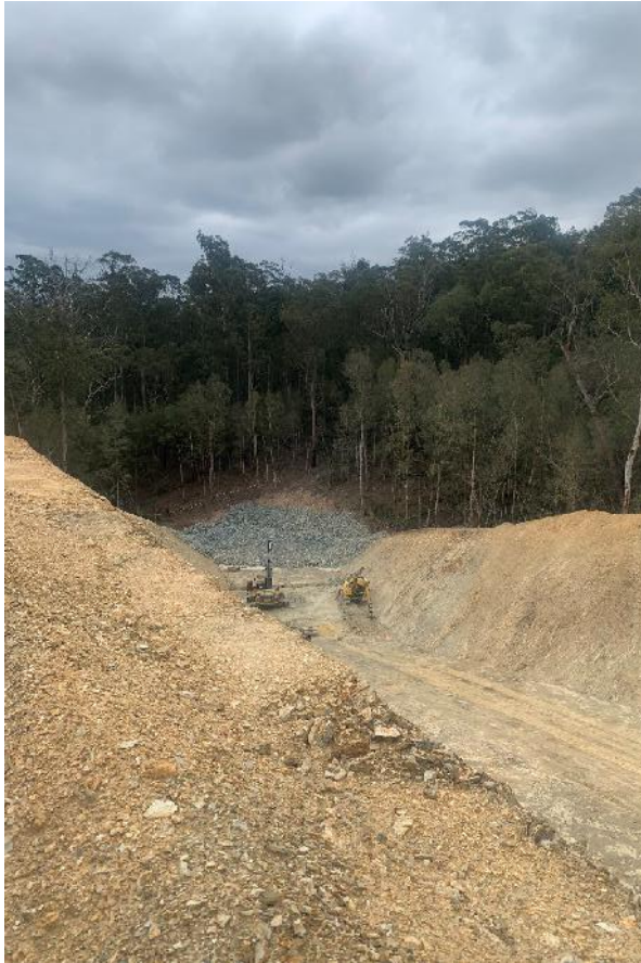
Spillway construction
