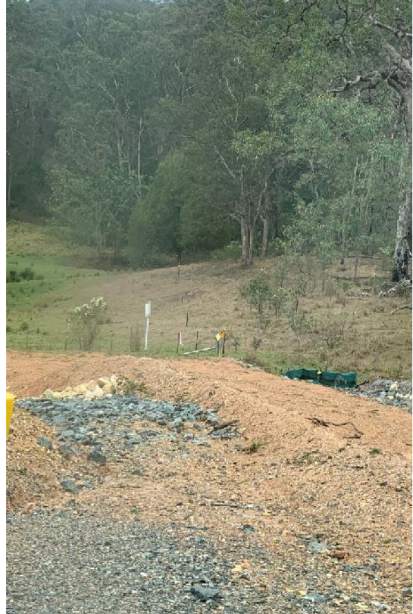
Dirty water drain into sediment basin (dry)
