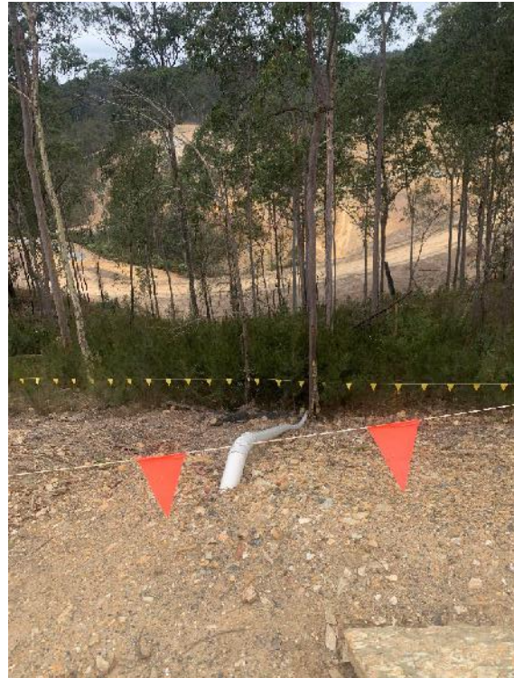
Sump by-pass pipe drains to the ground 15-NOV-2023 (defeating the purpose of the concrete-lined wash bay and associated sump)
