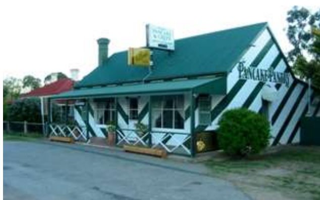
An example of inappropriate paint patterning on a historic building
