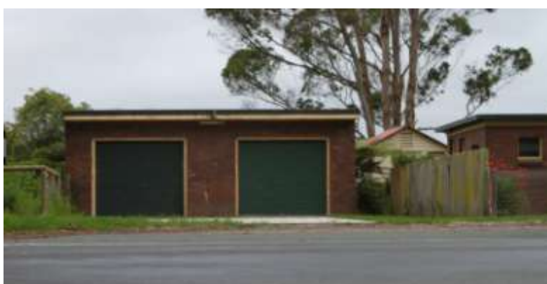
Police station garage
