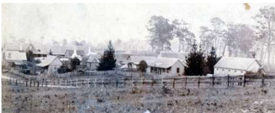
Bodalla circa 1885 looking to the north west from the approximate location of behind the present petrol station. The road in the foreground is not the highway, but joins it just off the right hand side of the photo, and runs across the south of the current buildings. The first Bodalla Hall can be seen on RHS of photo. All Saints Church is in the middle distance. Source: David Postill and Laurelle Pacey.
