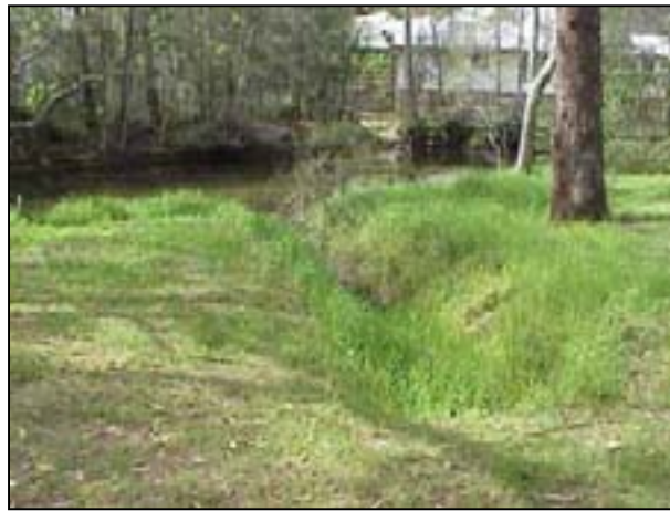
Figure 2-4 Stormwater pipe exit location at Highview Avenue
