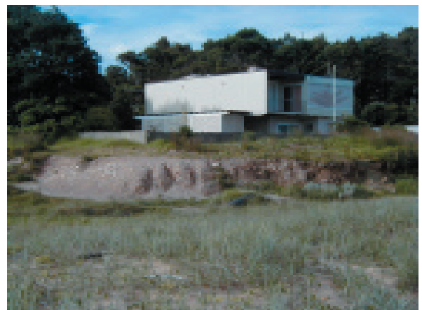
Plate 54: The creek outlet in the central part of the beach is very eroded and requires stabilisation to protect adjacent properties.
