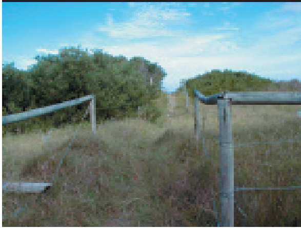
Plate 49: Over time, fences protecting the sensitive dunes have been vandalised or fallen into disrepair. They will need to be repaired and maintained in order to ensure the long-term success of dune stabilisation and revegetation works.
