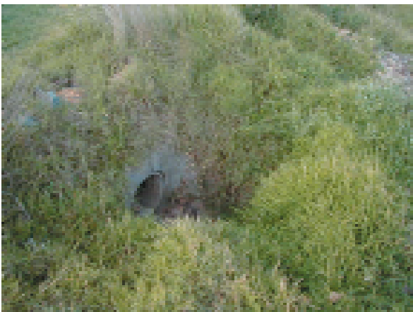
Plate 62: A drain outlet discharging stormwater just near the wetland. This discharged water receives no treatment before entering the Lagoon, despite the likelihood of high sediment loads and toxic particles from road runoff being contained in the water.
