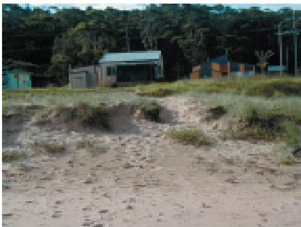
Plate 53: Dune vegetation has been largely cleared behind properties along Sandy Place, which has resulted in parts of the dune becoming unstable and being eroded. To prevent the same kind of damage, indigenous vegetation along the western section should be fenced and protected.
