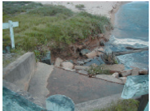
Plate 52: The culvert at Bay Road has become deteriorated. Flows after storms cause scouring and erosion to the beach.
