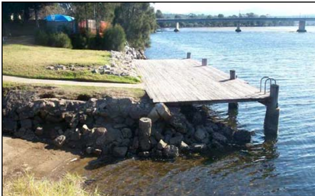
Photo 11: The Moruya Town Wharf and Boat Ramps
