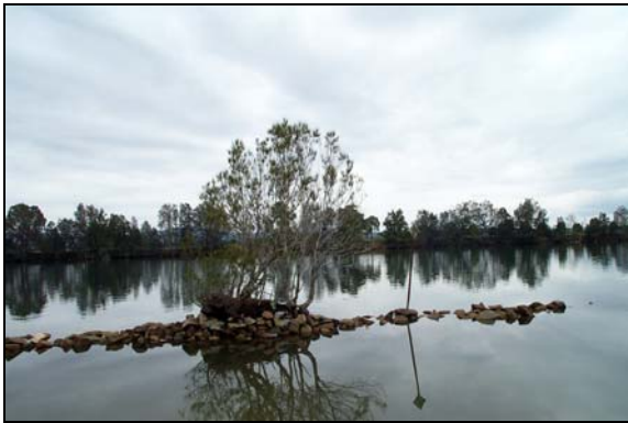
Photo 17: Casuarinas assisting with training wall stabilisation where Ryan's Creek meets the Moruya River.
