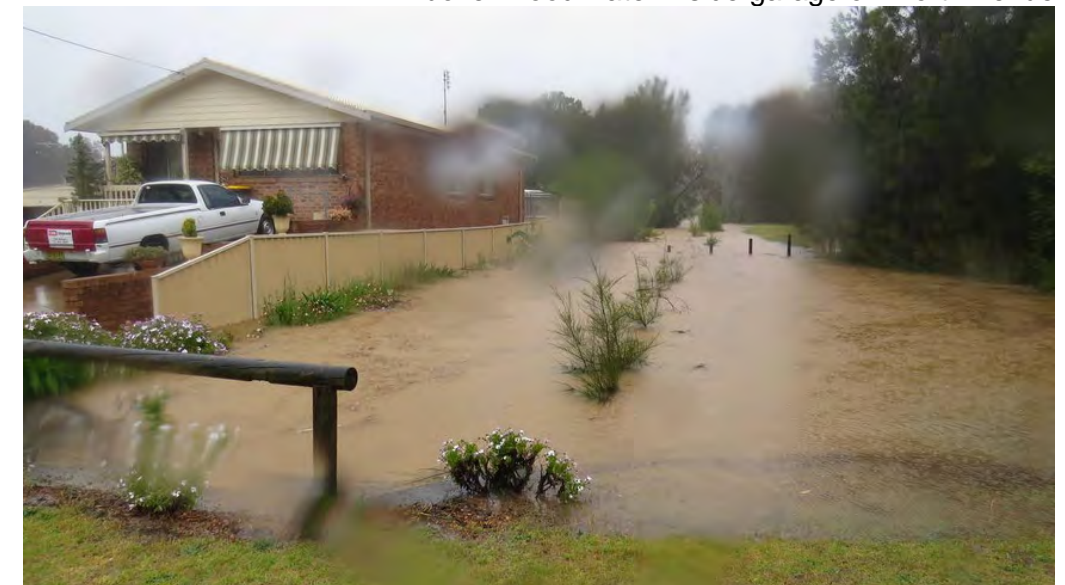
Above: Channel between Mort Avenue and Tatiara Street (upstream of Mort Avenue)
