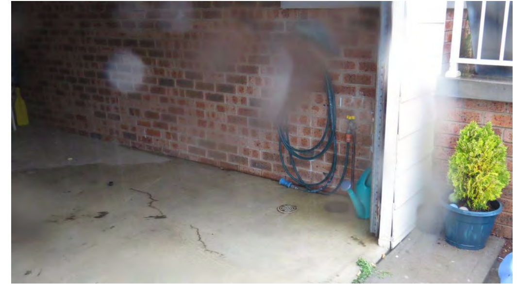
Above: Flood water inside garage on Mort Avenue
