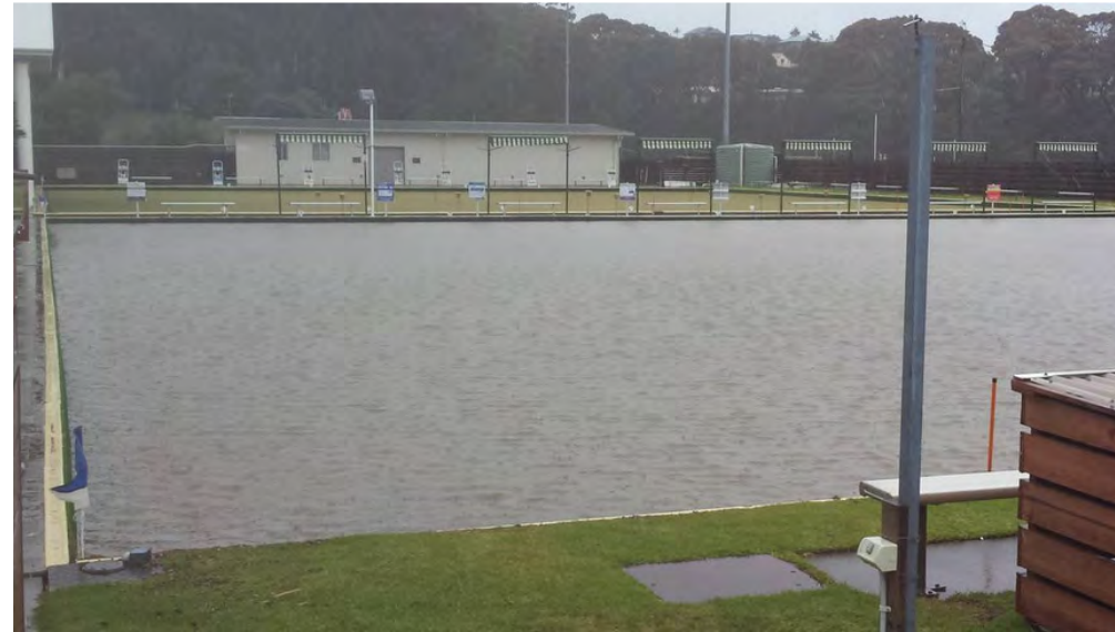
Above: Flooding of the Bowling Green
