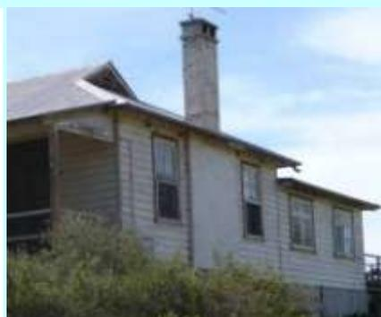
The gabled hip, vertical panelling in the verandah return, shiplap profile weatherboards, exposed rafter ends, protruding chimney back and separate roof to the rear rooms demonstrate how form and detail have been used to enrich the old school building.
