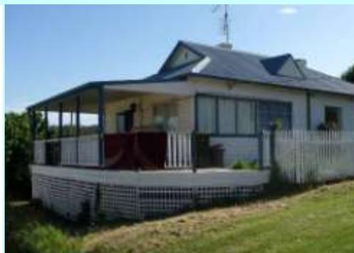
This adapted federation style cottage shows the use of weatherboards below the windows with cement sheet above. The new verandah is treated as a separate element and so reduces impact on the historic roofline.
