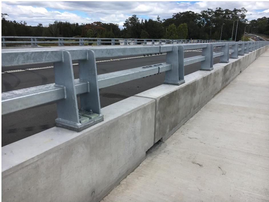
Example traffic barrier to shared pathway allowing protection and viewing from the roadway
