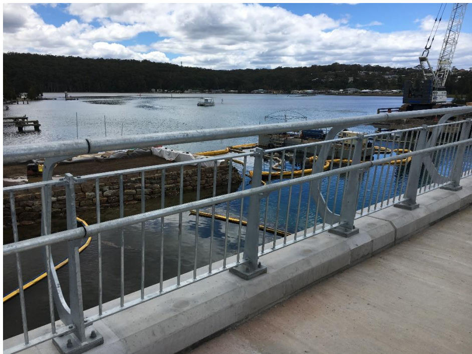
Example bridge railing system to a shared pathway with excellent viewing out for pedestrians
