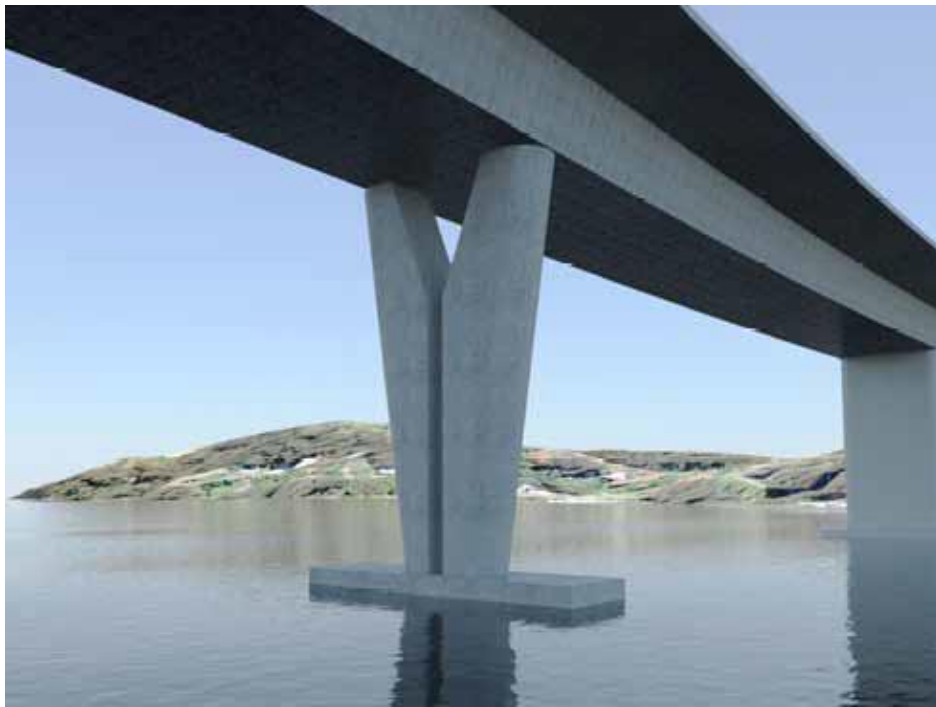
Example of the preferred V-shape pier arrangement as shown in the RMS documentation
