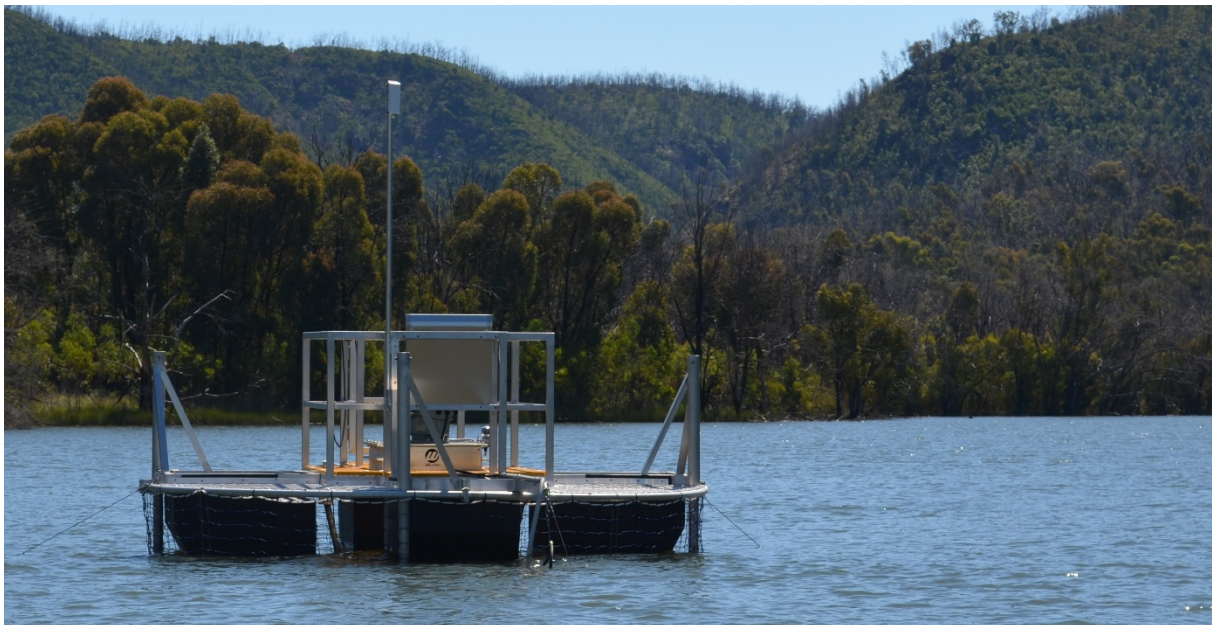
Figure 13.1: Example installation of ResMix3000 (Photo supplied by WEARS Australia)
