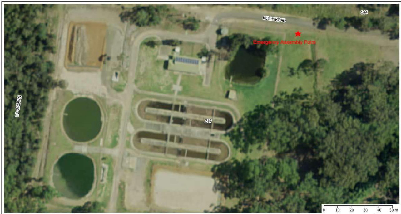
Figure 15 - 7: Tuross Head STP Emergency Evacuation Point
