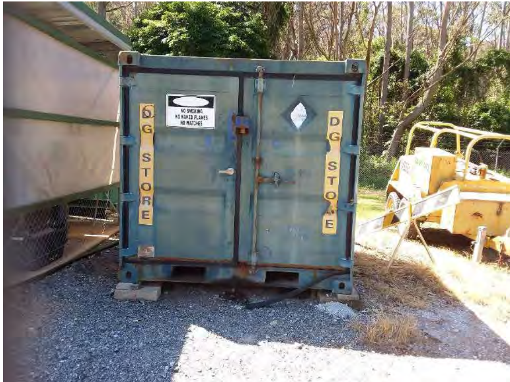
Figure 16 - 7: Narooma STP – Chemical Storage Container
