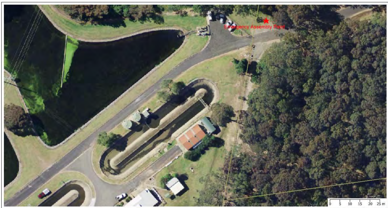
Figure 16 - 9: Narooma STP Emergency Evacuation Point
