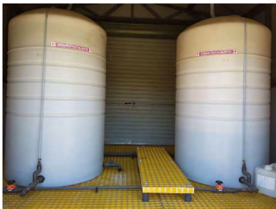
Figure 14 - 7: Moruya STP – Chemical Storage Sodium Hypochlorite
