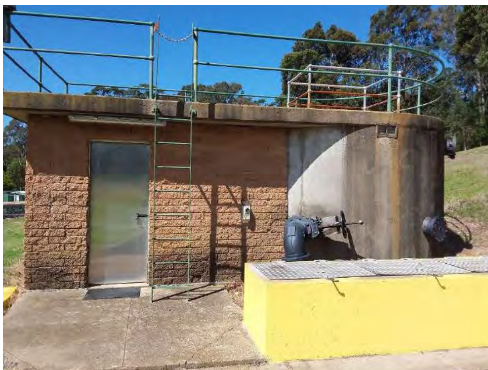
Figure 16 - 8: Tomakin STP Inflow Balance Tank and Channel
