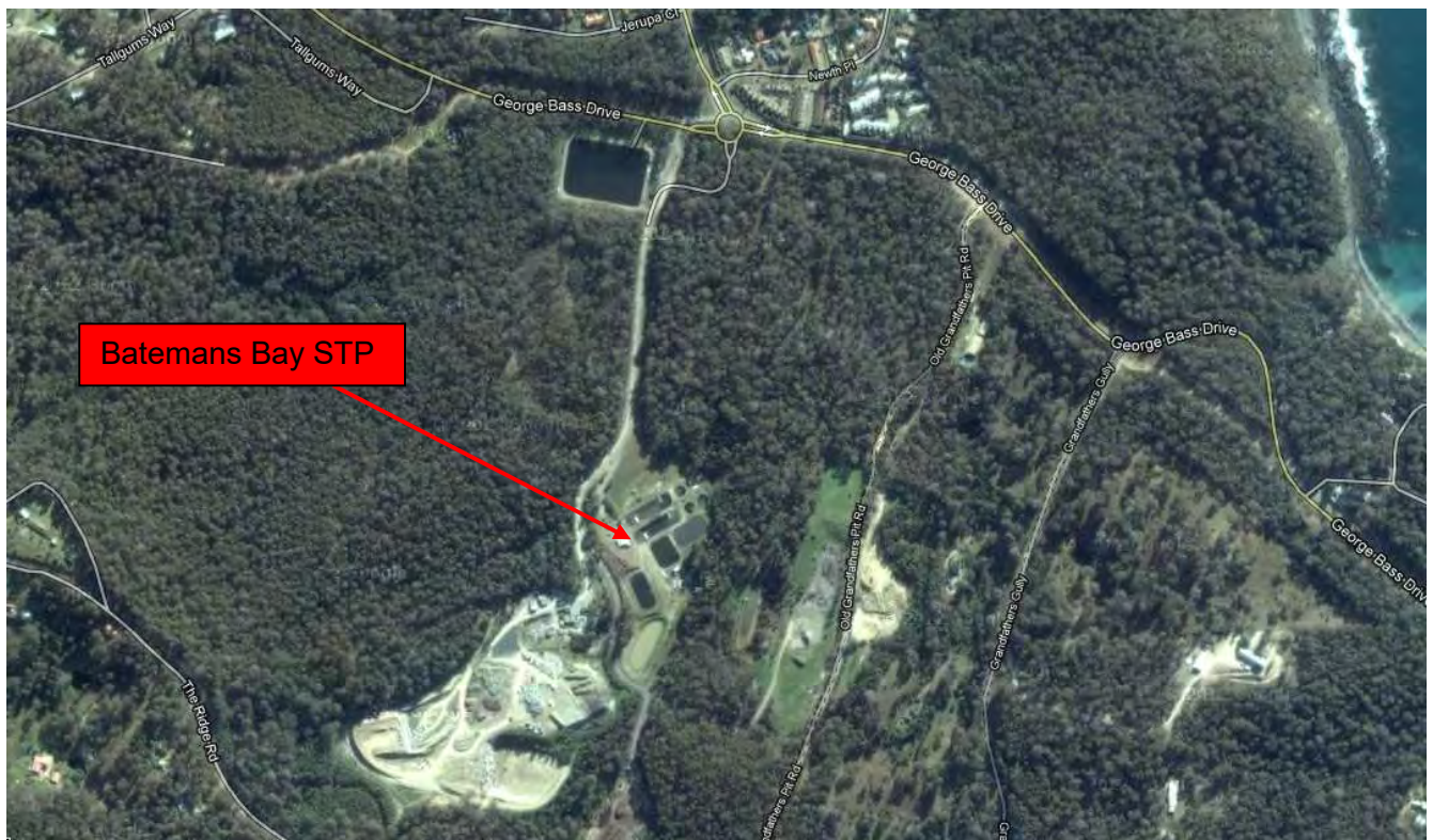
Figure 12 - 1: Batemans Bay STP Location
