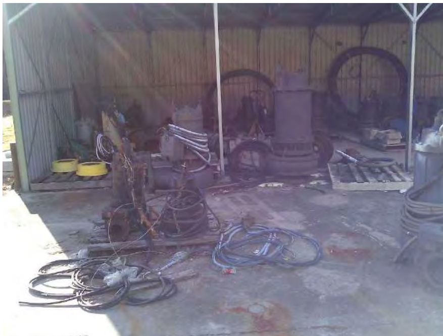
Figure 6 - 7: Spare Pumps Stored at Tomakin STP
