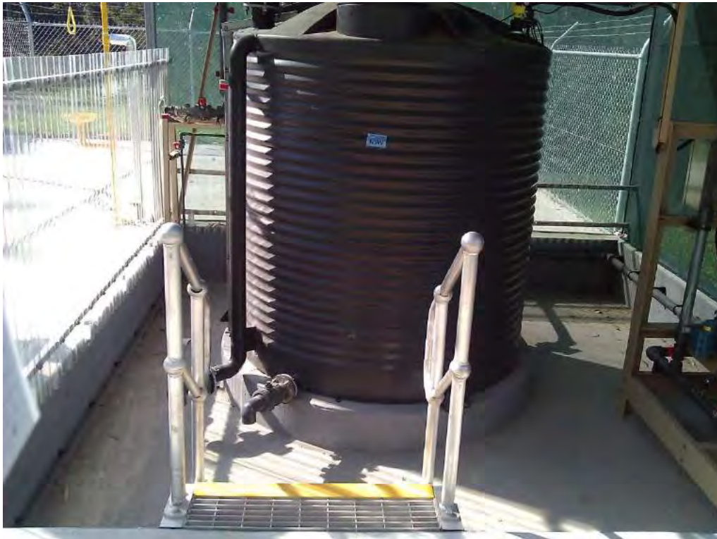
Figure 6 - 9: Typical Chemical Storage Container for ESC's STPs
