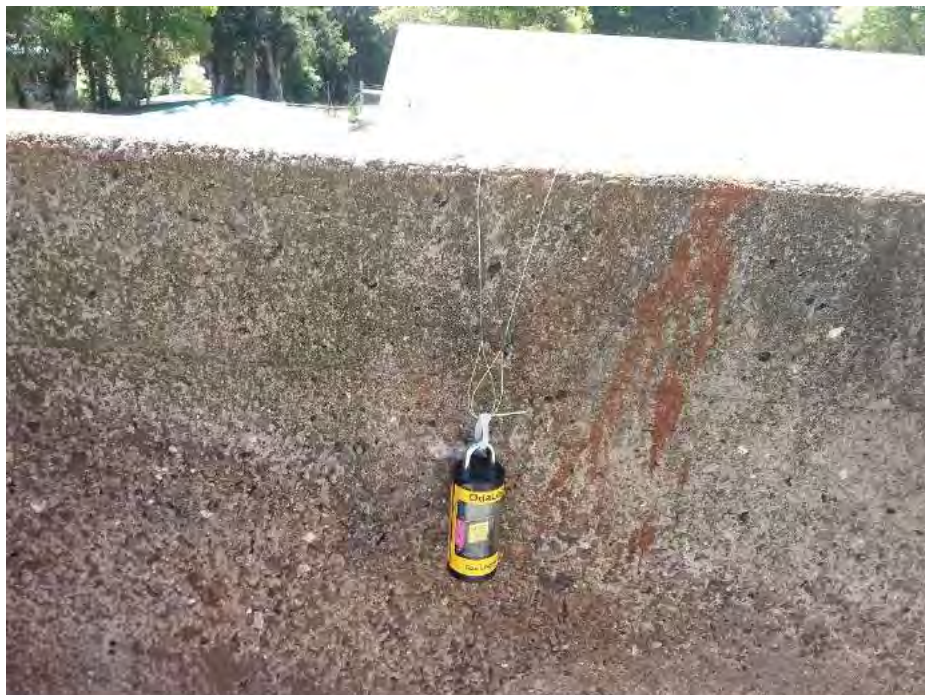
Figure 13 - 5: H 2 S Monitor Used in the Tomakin STP
