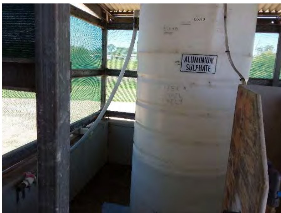
Figure 14 - 5: Moruya STP – Chemical Storage Alum Sulphate Used for Effluent Reuse
