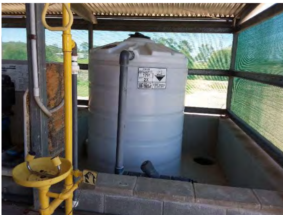
Figure 14 - 5: Moruya STP – Chemical Storage Alum Sulphate Used for Effluent Reuse
