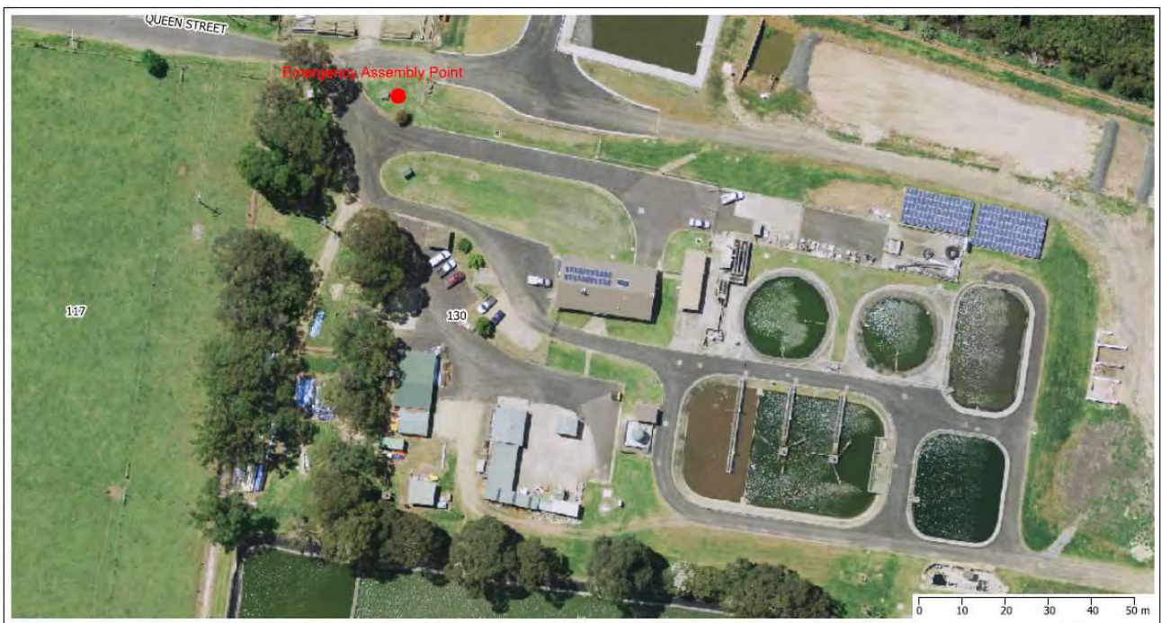
Figure 14 - 8: Moruya STP Emergency Evacuation Point
