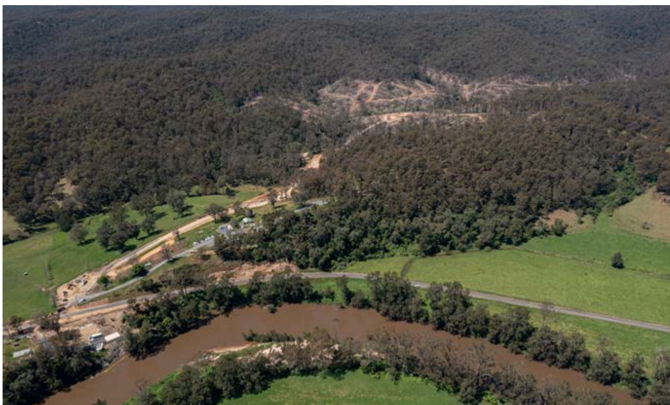
Image: Construction of the new southern dam, west of Bodalla, is on track.
