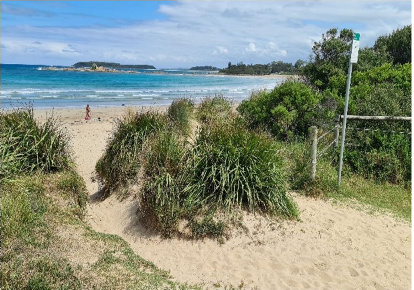
Kingston Place Entrance February 23 – Where the stairs were removed after storm damage.
