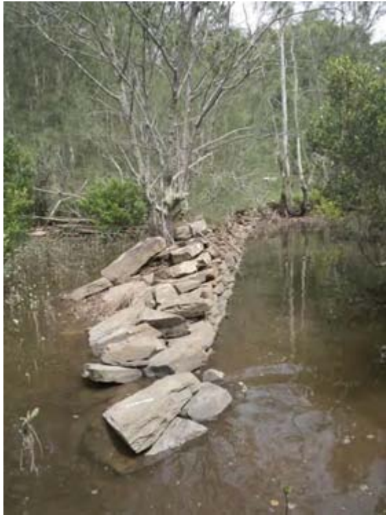
Stone wall taken from the east, note how it is keyed into the western bank with stones.
