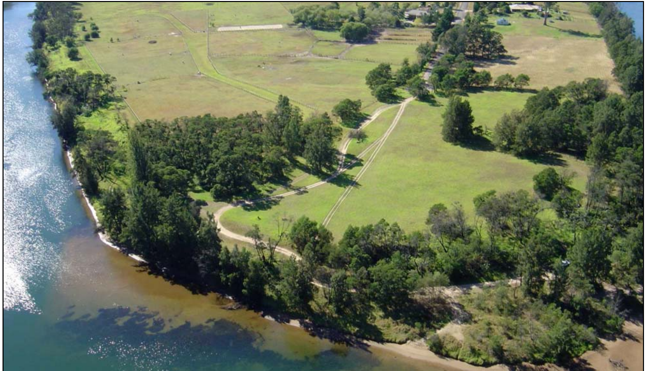
Figure 4 Aerial Photograph illustrating the gravel access tracks through the reserve (April 2006)
