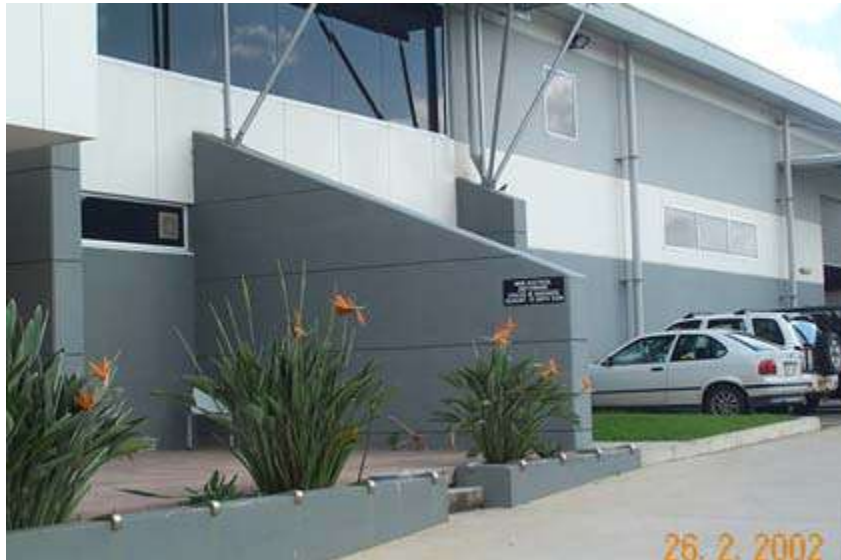
Fin walls obstruct sightlines and create concealment spaces
