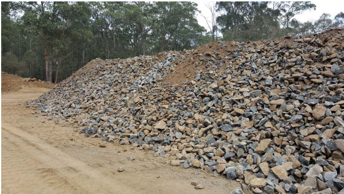
Figure 8: Rockfill stockpile at Bay Sand and Gravel 20/1/17
