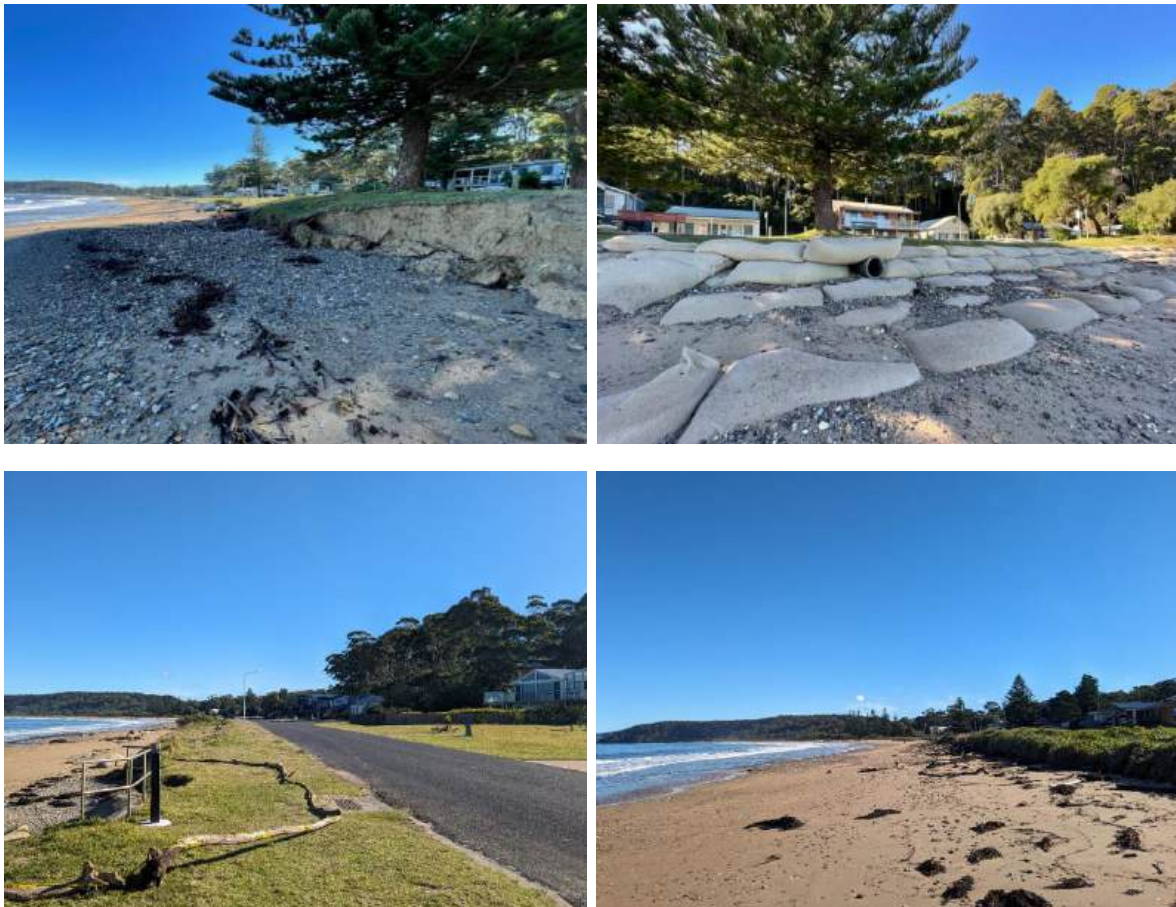
Figure 1-2 Images of coastal erosion and infrastructure at the site (Worley, 2024)
