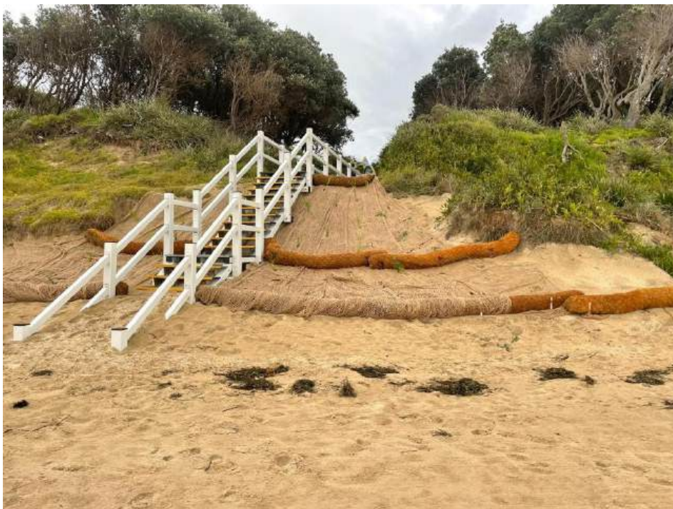
Figure 3-4 Example FRP beach access stairs at Currarong (Worley, 2025)
