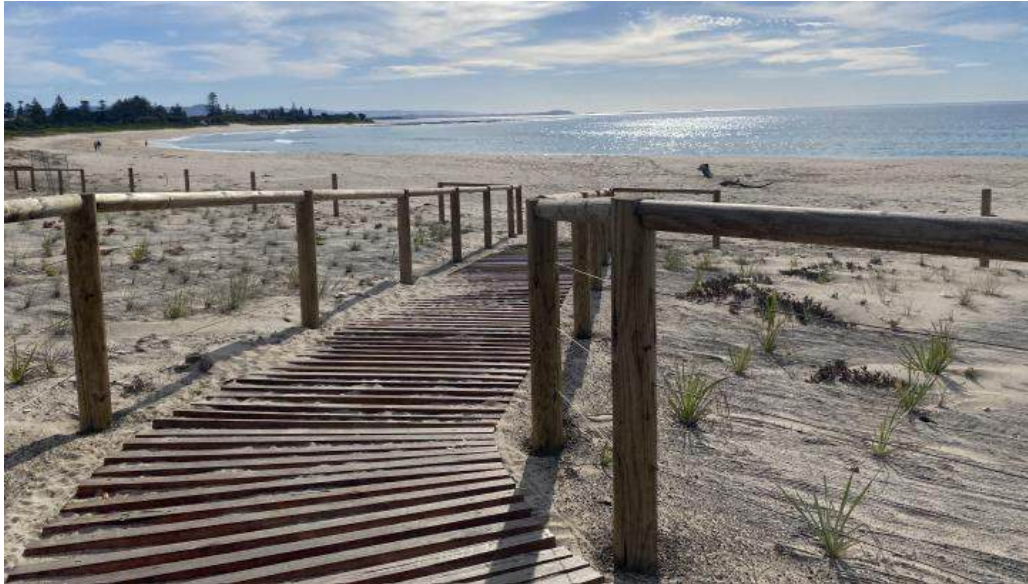
Figure 3-3 Example board and chain beach accessway Shell Cove (Worley, 2025)
