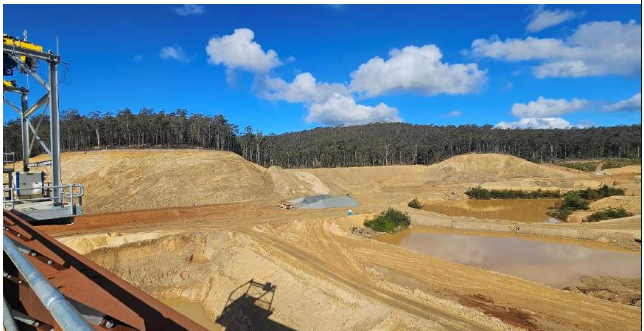
Plate 4 Construction footprint facing east from Tower Access Bridge: Sediment basin, and former borrow-pit,
