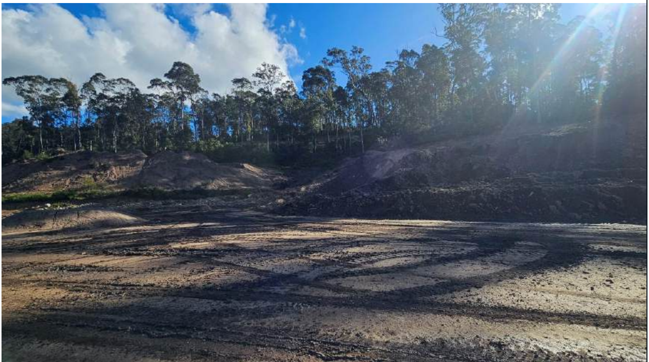
Plate 12 Topsoil storage upstream of water storage embankment facing west
