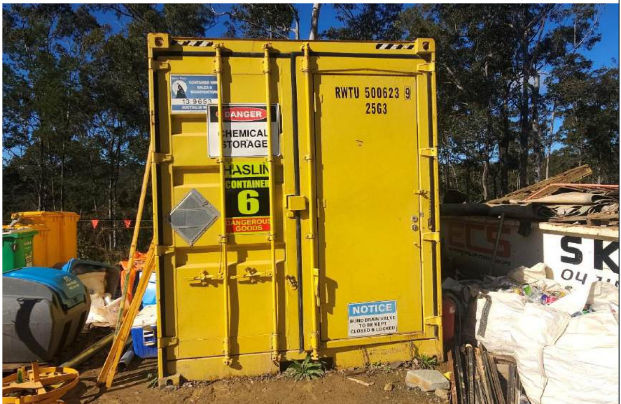
Plate 3 Self-bunded fuel and chemical storage at site compound
