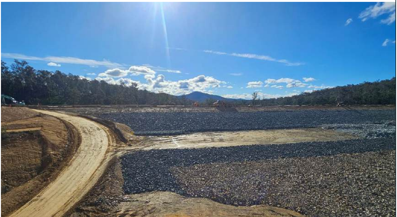
Plate.8 Construction footprint facing north-west from Tower Access Bridge: Water storage embankment
