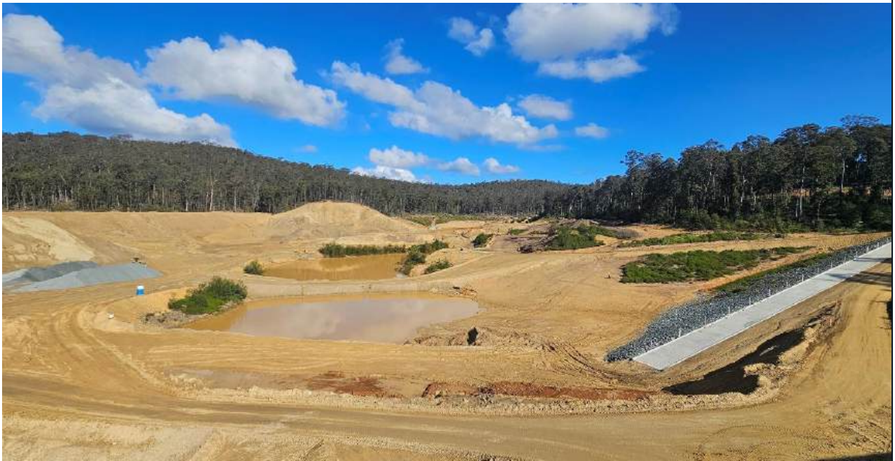
Plate 5 Construction footprint facing south from Tower Access Bridge: Sediment basin, topsoil storage, and boat ramp
