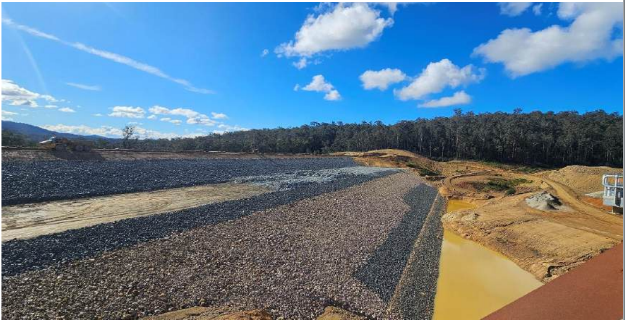
Plate 7 Construction footprint facing north from Tower Access Bridge: Water storage embankment, sediment basin, and spillway
