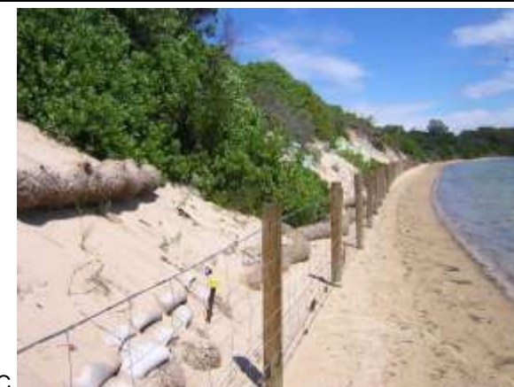
Figure 70: A - Signage installed at Tomakin spit, B – fencing on ocean side and dune crest (looking south), C – fencing on ocean side looking north
