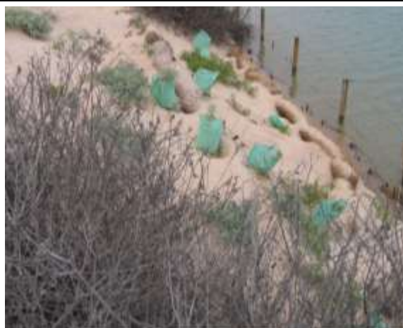
Figure 71: Coir log terrace, original fence and revegetation at Tomakin Spit
