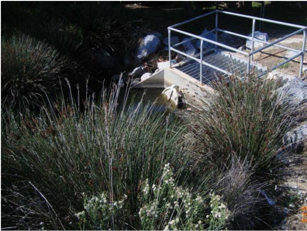
Figure 3.27 – GPT blocked by rubbish behind southern caravan park at Corrigans Beach (March 16 th 2010)
