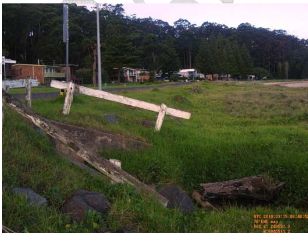
Figure 3.10 – Stormwater outlet protected by a buried rock seawall in front of Fauna Avenue at Long Beach (March 15 th 2010)
