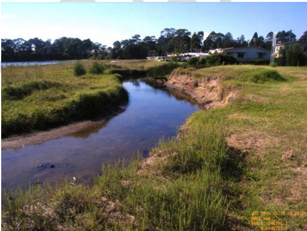
Figure 3.26 – Erosion of creek along the low-lying caravan park at the southern end of Corrigans Beach (March 16 th 2010)
