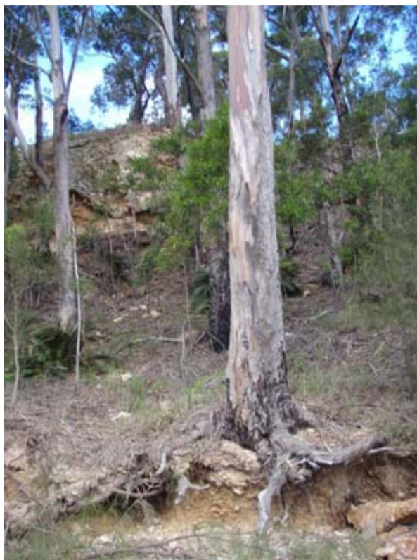
Figure 3.9 – Undercutting due to wave action at the bottom of a very steep slope east of Long Beach (March 15 th 2010)
