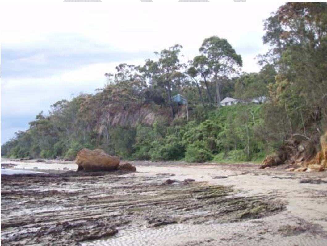
Figure 3.12 – Houses located at the edge of the cliff between Long and Maloneys Beach (March 15 th 2010)
