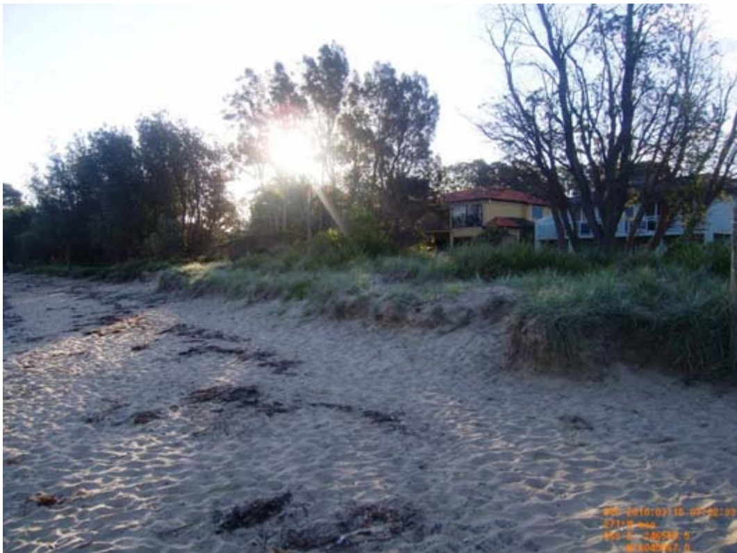
Figure 3.15 – Low-lying houses close to the eroding dune at the eastern end of Surfside Beach (March 15 th 2010)
