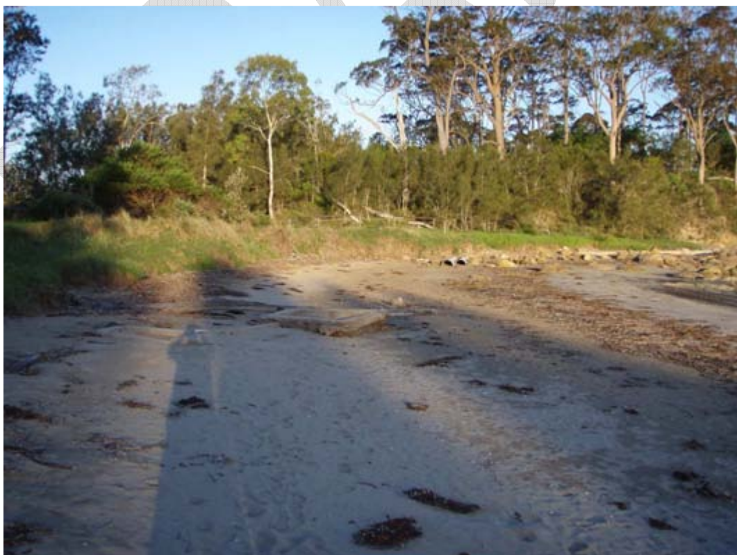
Figure 3.16 – Damaged stormwater pipe at Surfside Beach (March 15 th 2010)
