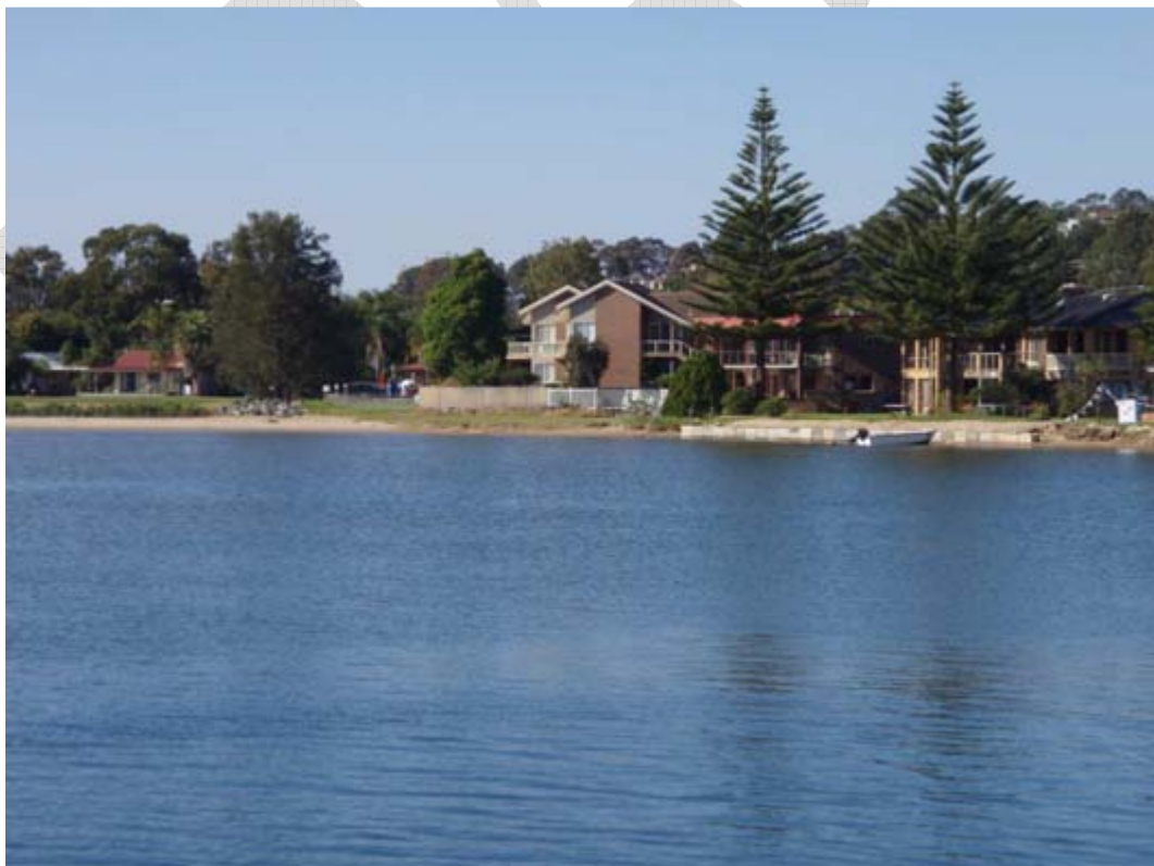
Figure 3.22 – Varying condition of seawall and unprotected low-lying houses within Batemans Bay Marina (March 16 th 2010)
