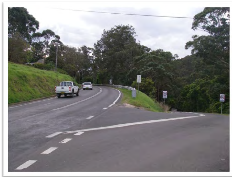
Princes Highway Near Centenary Drive – Note the Steep Fill Batter on the Right (east) and the Steep Cut Embankment on the Left (west).
