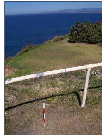
Low-profile barriers are usually a more continuous feature, but are also not a deterring or effective physical barrier.
