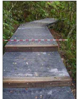
On-ground fiberglass mesh boardwalks, on timber or recycled plastic framework, in simple and more sophisticated designs (left and right).
