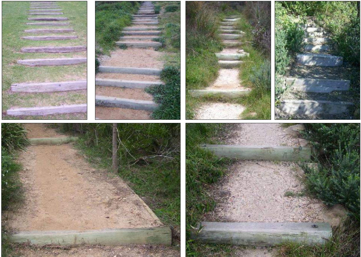
Examples of embedded sleepers on a gentle slope (top left), timber edged step-and-runs (top centre) and flat-set timber treads (top right). Examples of boxed timber steps and retaining toe stones (below), with compacted gravel backfill..
