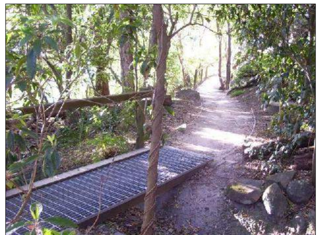
Low-key track bridge, with timber frame and expanded fibreglass decking.
