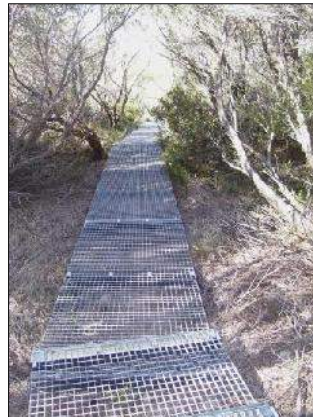
On-ground fiberglass mesh boardwalks, on timber or recycled plastic framework, in simple and more sophisticated designs (left and right).
