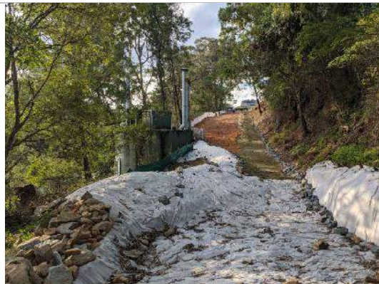
Figure 4-6 Vehicle access track. Sump installed at hydraulic low point. Sediment fence erected on western edge and dirty water drain runs along eastern edge.
