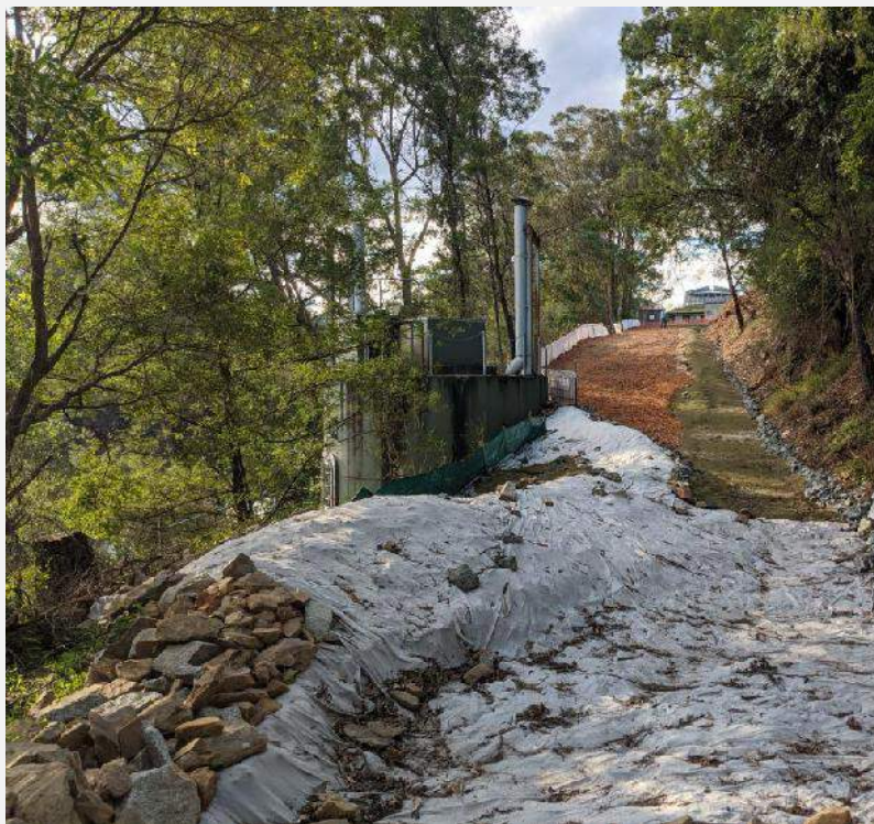
Figure 1. Post TRIPS Stage 1 vegetation clearing and ERSED controls
