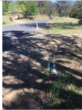
Figure 4-3 Driveway entrance to TRIPs site. Existing PVC pipe culvert (blocked)
