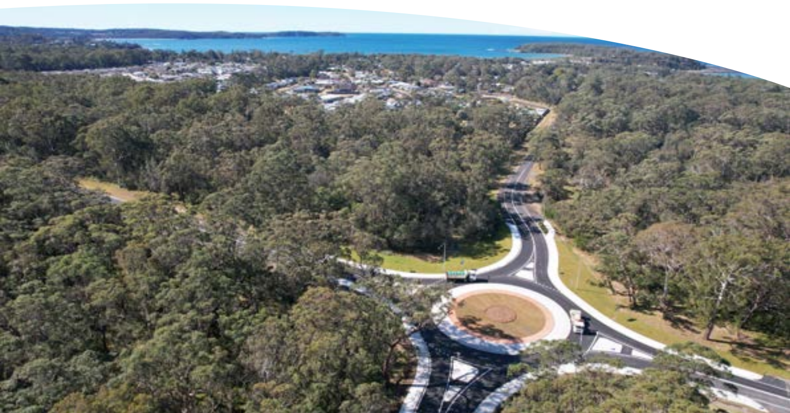
Image: This intersection on busy George Bass Drive was realigned and a roundabout constructed.
