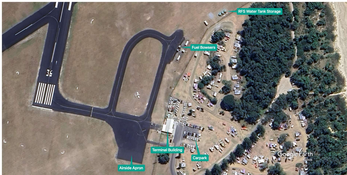
Figure 26: Terminal Precinct Aerial Image
