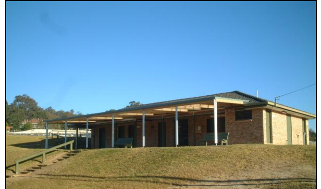
Dalmeny Oval Facilities Building
