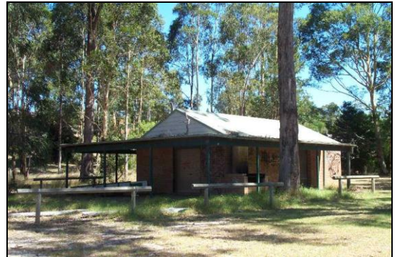
Surf Beach Amenities Building
