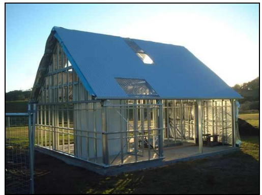
Tilba Amenities Building Under construction August 2006
