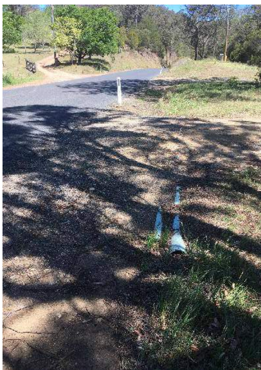
Photo 2-2. Driveway entrance to TRIPS site. Existing PVC pipe culvert (blocked)
