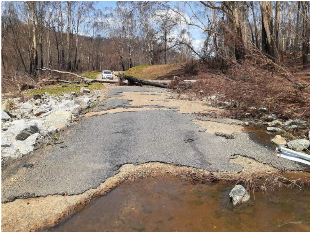
Photo 15 – part of the southern causeway Gulph Creek Eurobodalla Road, Nerrigundah. This photo highlights the devastating impact of both the bushfires followed by a natural disaster flood event.
