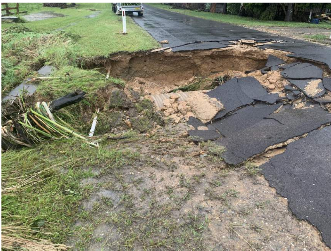
Photo 16 Veitch Street, Mogo – culvert crossing December 2022 was restored that evening and re-opened to provide resident access. Major renewal/replacement will be required in the short term.
