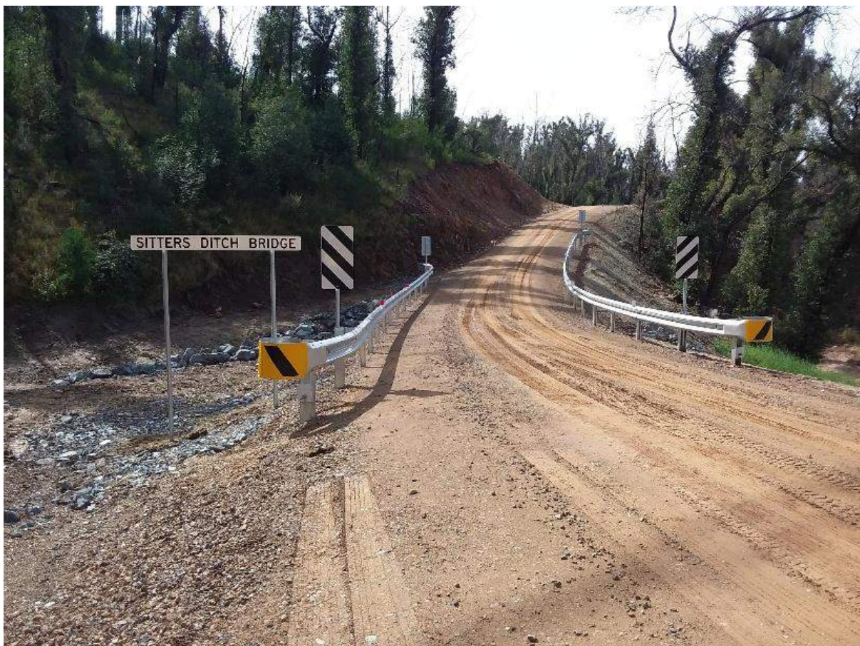
Photo A.26 – Sitters Ditch bridge The bridge was replaced with a multiple cell concrete culvert
