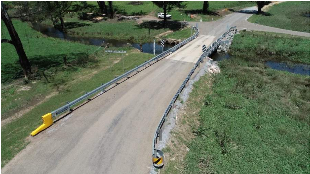
Photo A.5 – Cheese Factory bridge was replaced with a new concrete bridge
