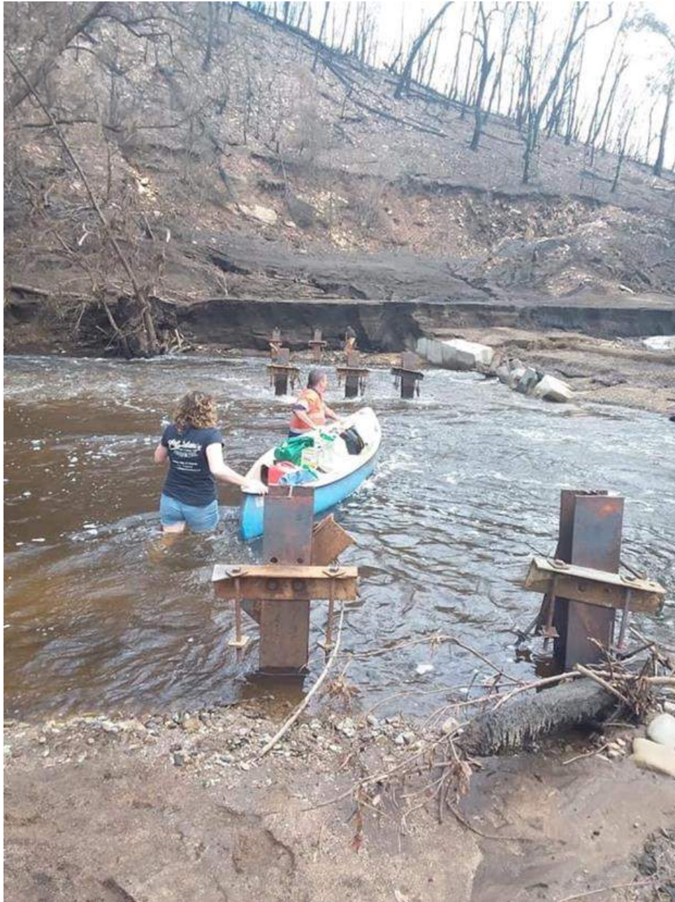
Photo 13 – significant challenges face rural farmers and residents when critical infrastructure is lost. Belimbla bridge was destroyed on 31 December 2019. Temporary structures suffered repeated damage during subsequent repeat flood events
