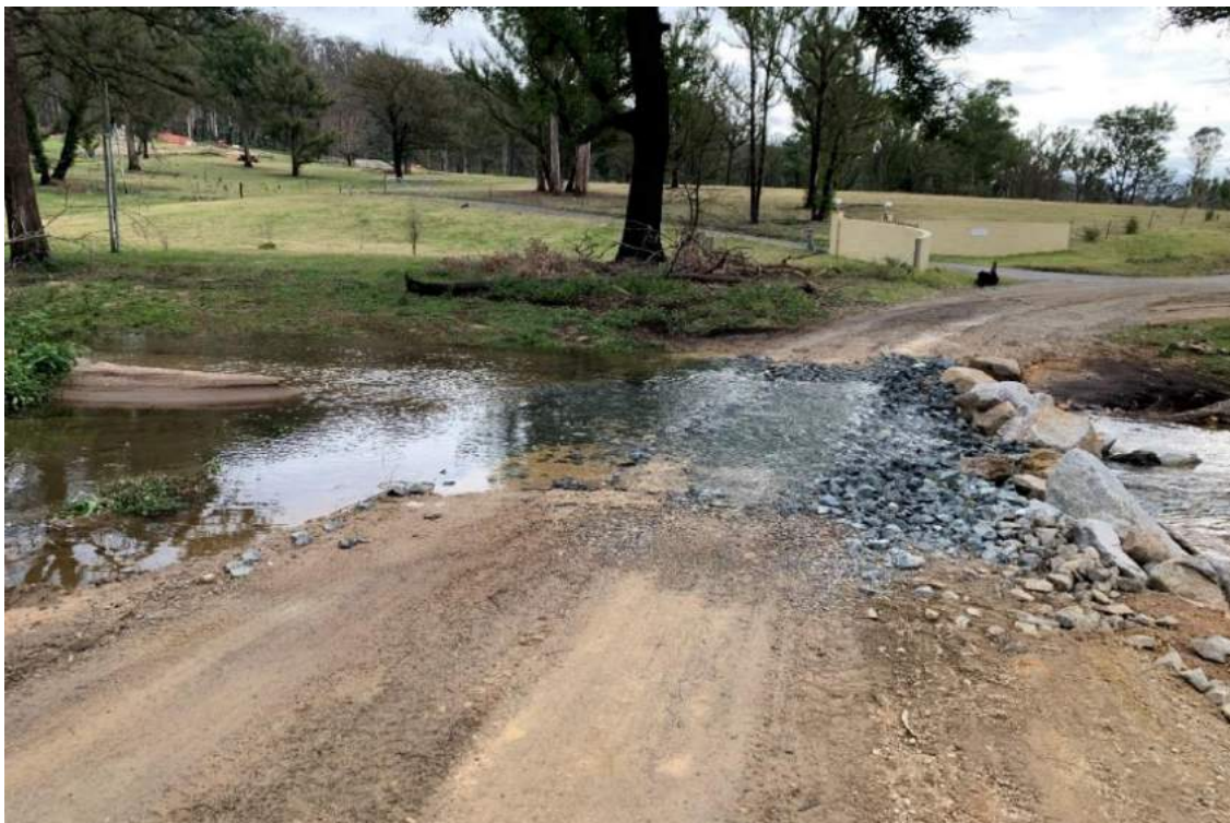
Photo 17 - Nelligen Creek Road causeway has been repeatedly washed away
