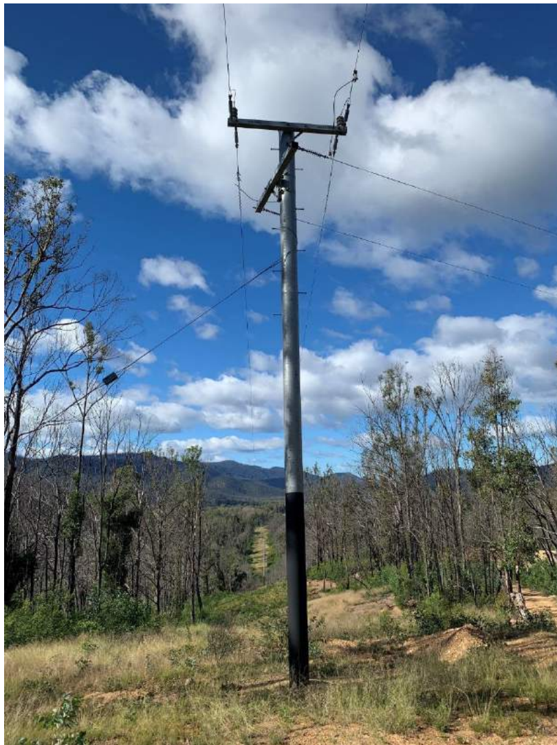
Photo 22 – resilient power poles survived the intense bushfire at Merricumbene. Broader application would significantly improve the resilience of the power supply network.
