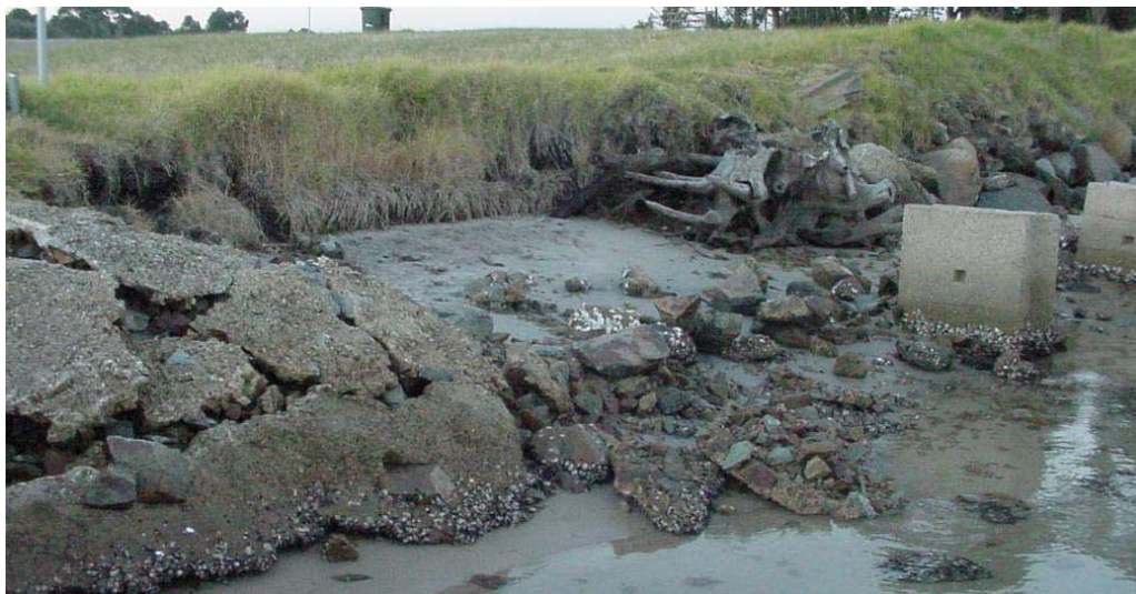
Figure 17: Bank erosion behind the rock riprap. Bank erosion behind the rock riprap lining was observed in a number of places.
