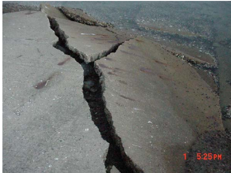
Figure 15: Infrastructure damage caused by erosion.
