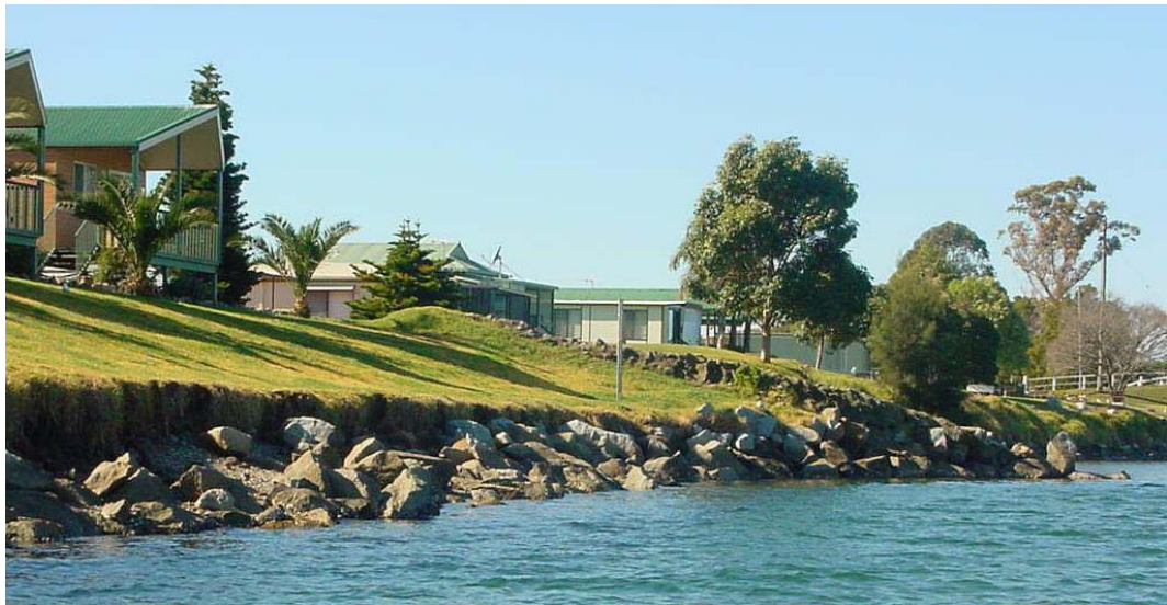
Figure 18: Vertical banks subject to bank erosion at the rear of the motel.
