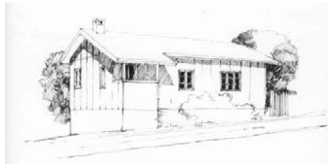
3. Gable roofed cottage with fibre cement flat sheet cladding. Wall lining sheets and cover battens are set out to match window openings. Overhanging gables give some weather protection to end walls. Roof is extended to form a sheltering entry porch. Fibre cement roof.
