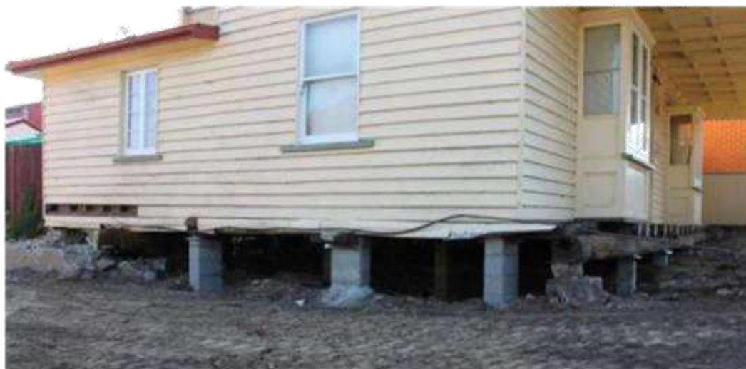
Funded work of restumping and levelling completed
