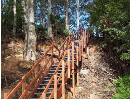
Stairway connecting Corrigan's Beach to Observation Point
