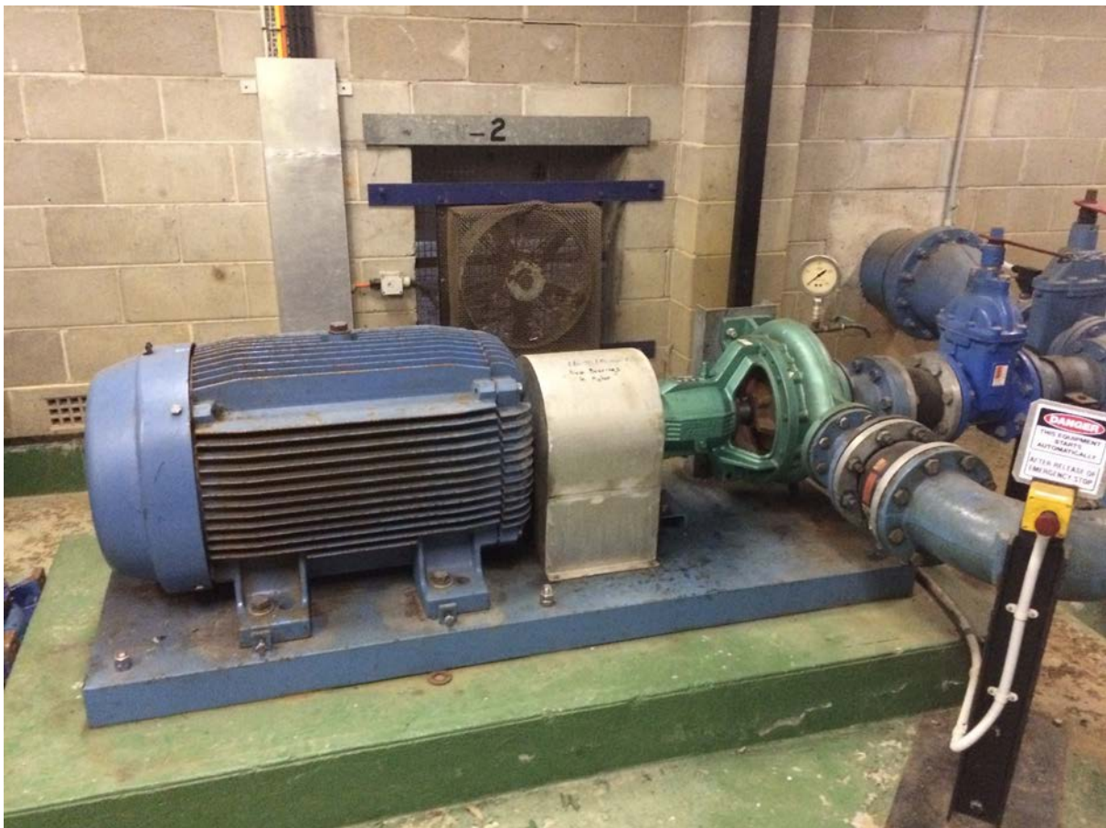
Figure 8- Existing Transfer Pump
