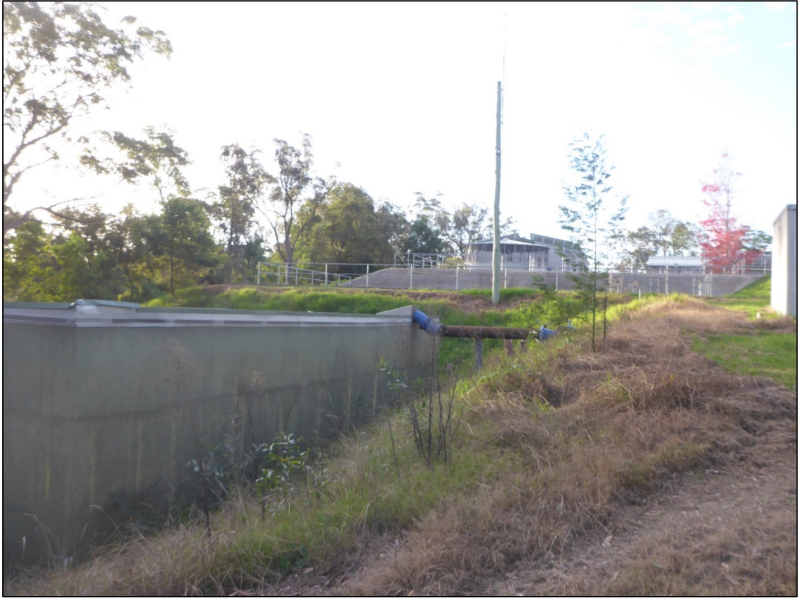
Figure 7- Existing Southern WTP clear water reservoir
