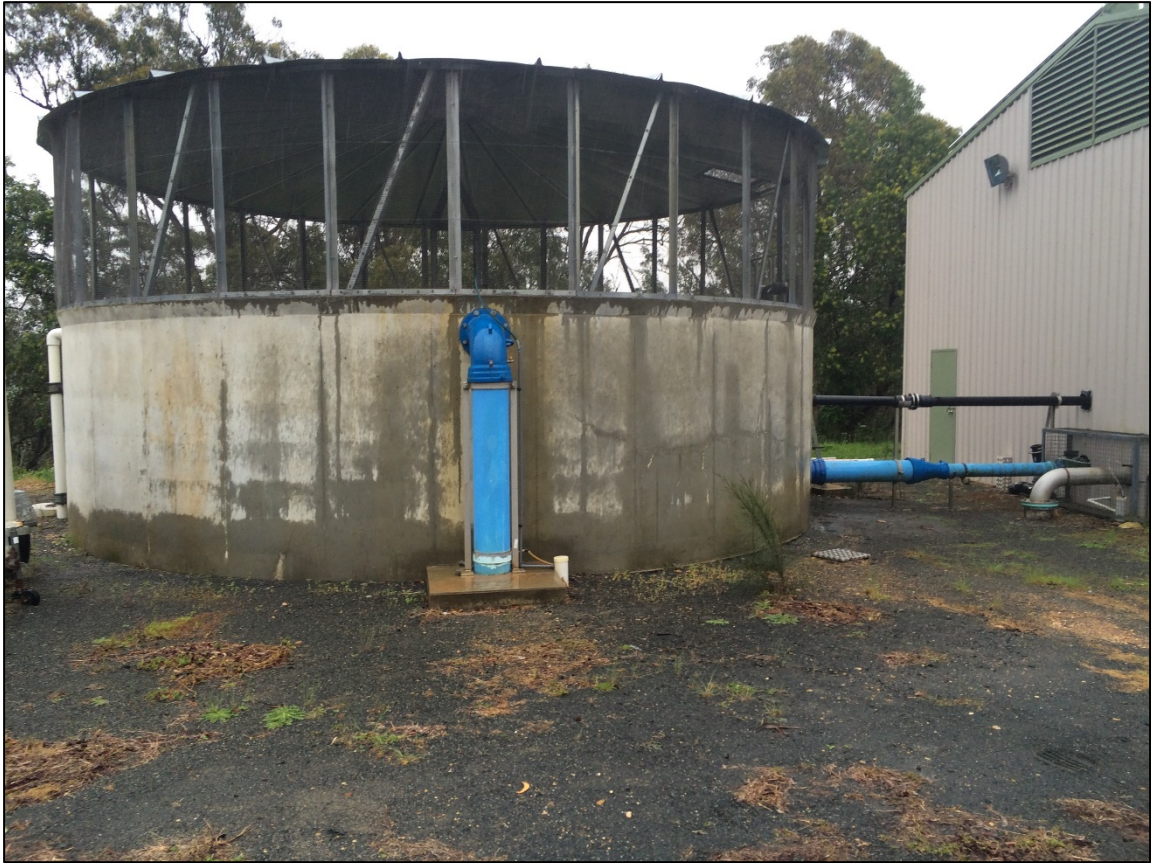
Figure 6- Existing Southern WTP Balance Tank
