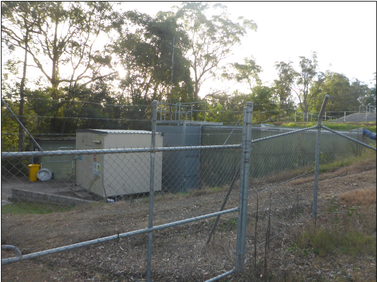
Figure 5- Existing Southern WTP clean water tank
