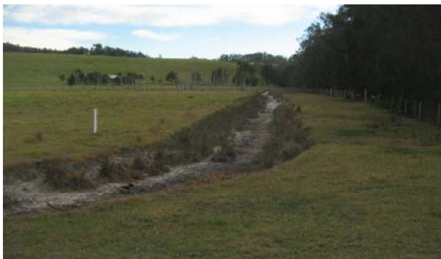
Figure 2-1 Constructed drainage channel in lowest lying private lands adjacent to Coila Ck
