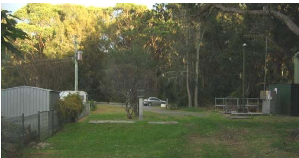
Figure 2-4 Sewage pumping station behind Lakeside Drive properties, Kianga
