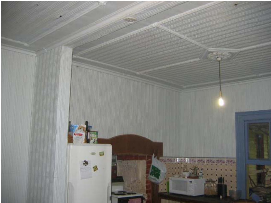
View of the opening that was formed when the rear bedroom was adapted to become a kitchen.
