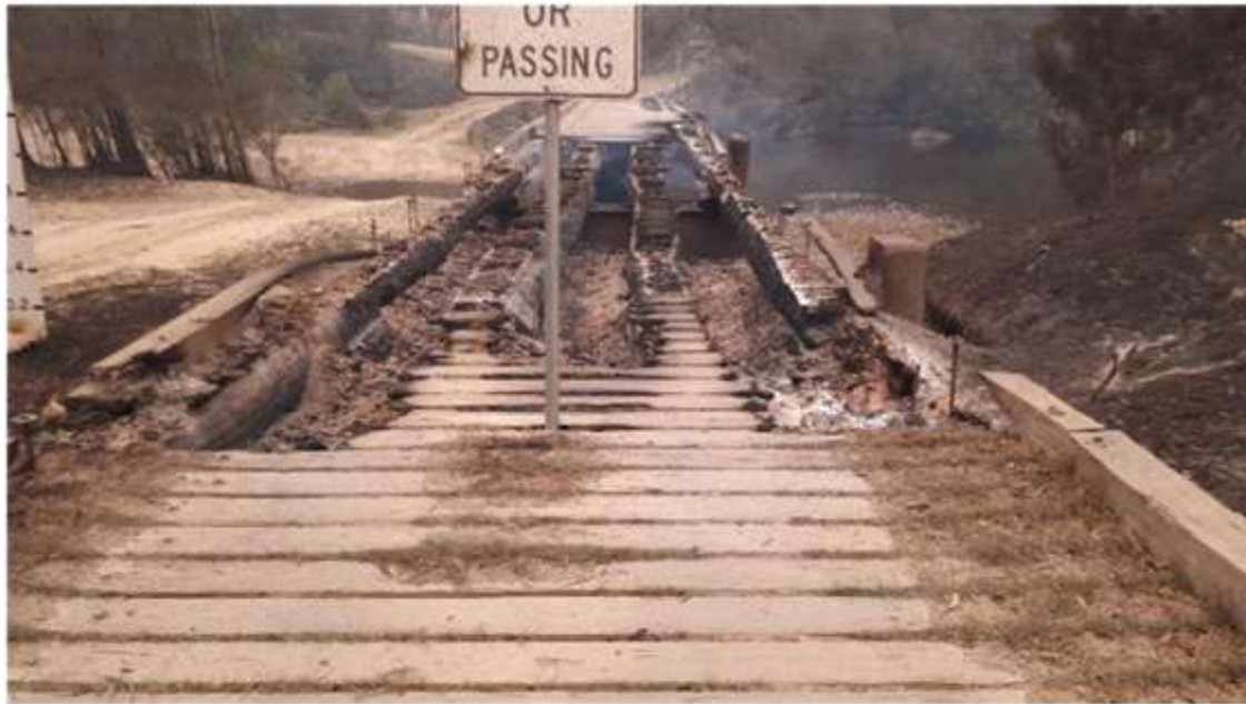
View from southern abutment
