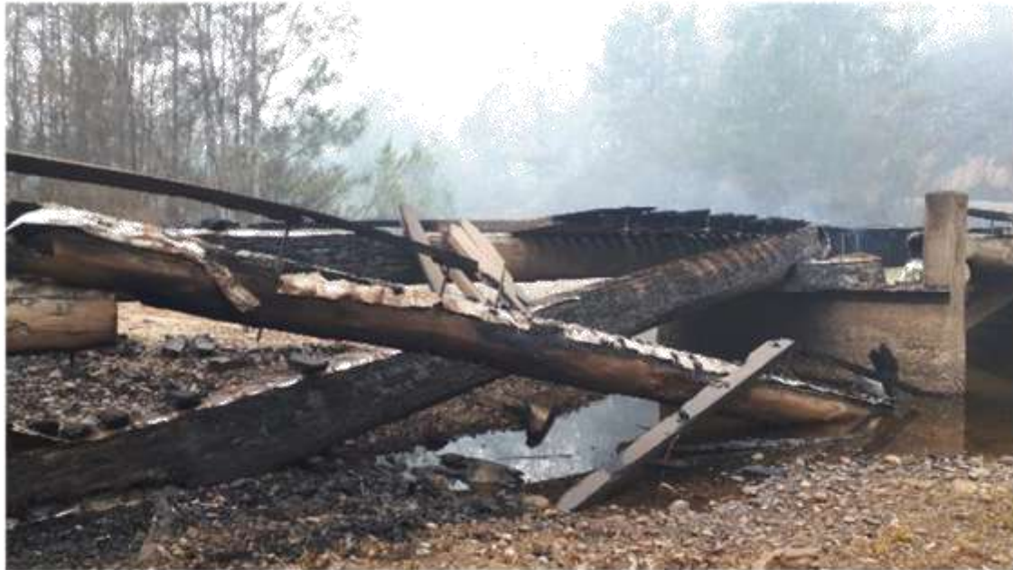
View from northern abutment
