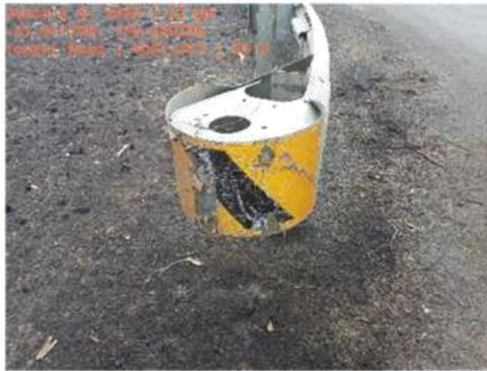
Yowani Road (Rosedale) guard rail damaged
