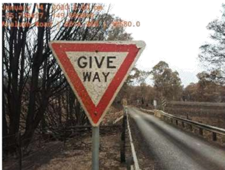
Fire damaged 'Giveaway' sign along Araluen Road
