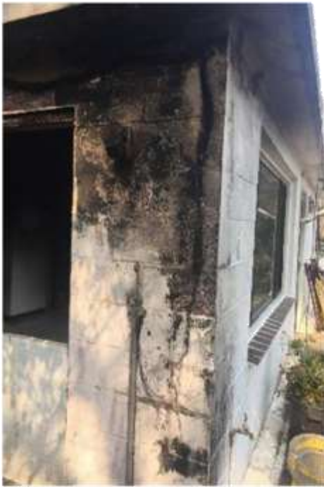
Example of destroyed control panel
