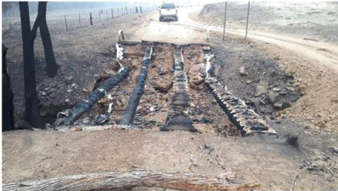
Four Gums Bridge
