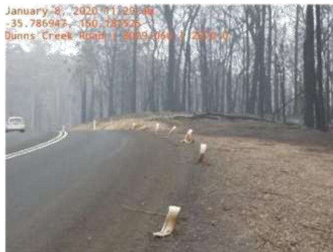
Fire damaged Guide posts along Dunns creek road (Tomakin)
