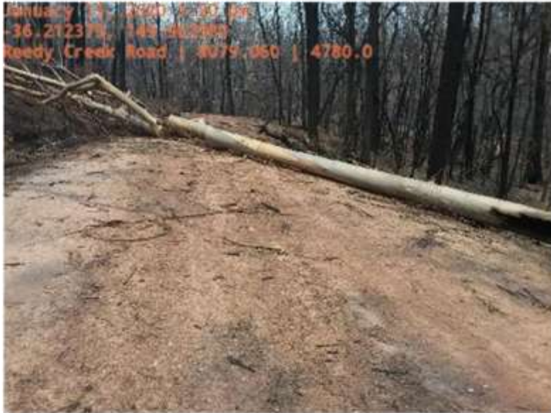
Reedy creek road, tree vegetation on road
