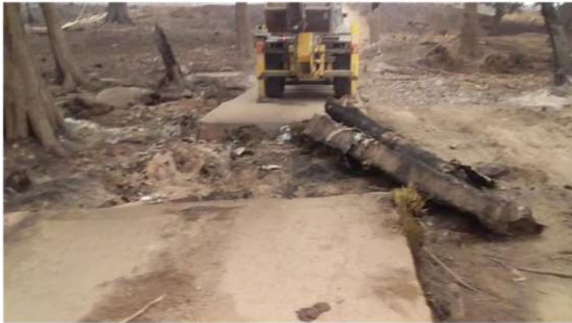
Johnsons Crossings Causeway
