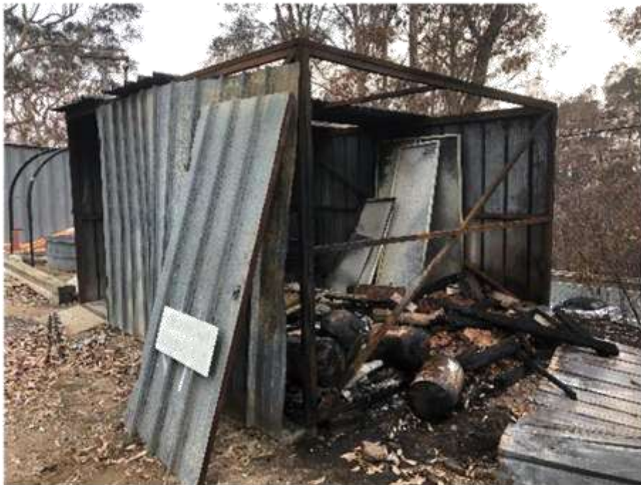
Shed in Batemans Bay Depot
