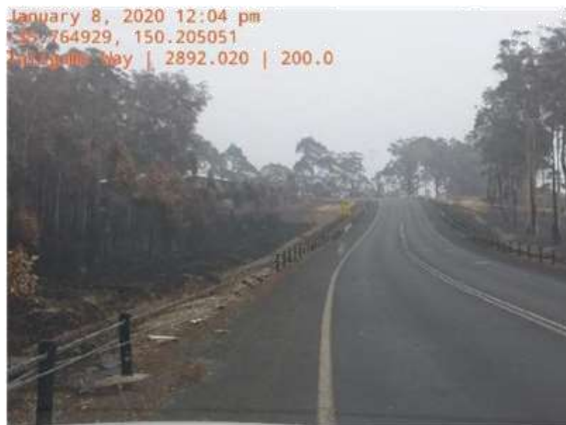
Protective Fence damaged from falling tree along Tallgums way (Surf Beach)
