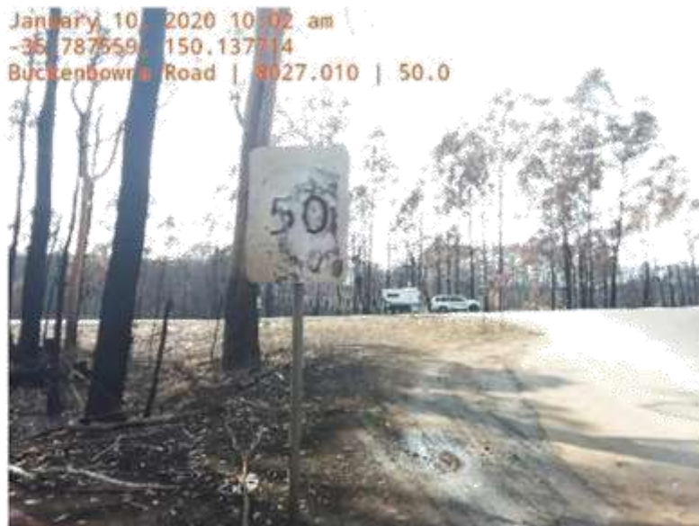
Fire damaged 50km/h sign on Buckenbowra road (Buckenbowra)
