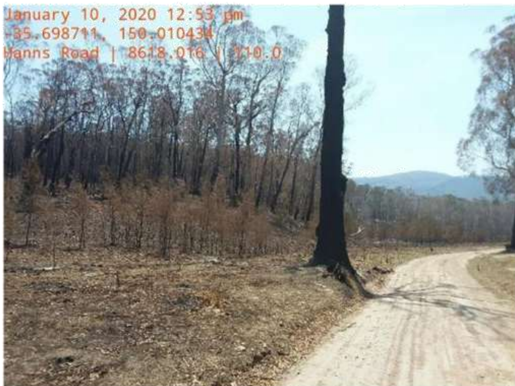
Hanns road, overhanging fire damaged tree along road side
