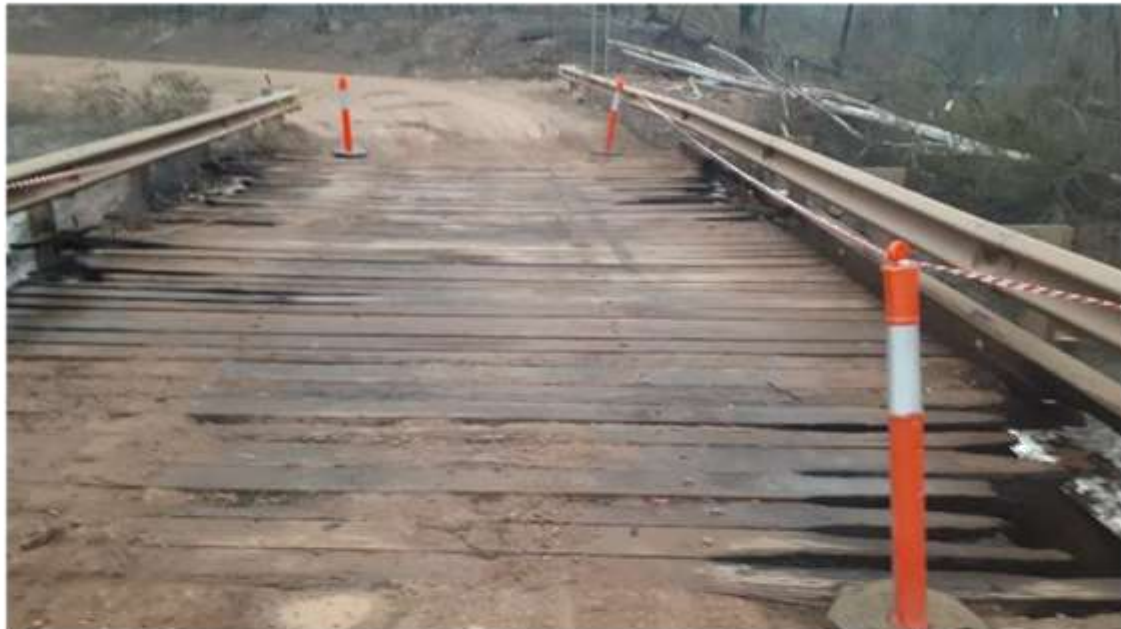
Kennys Creek Bridge
