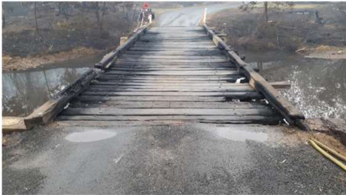
Gulph Creek Bridge
