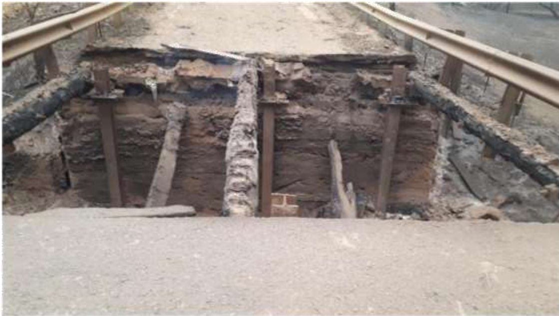
Pigeon Gully Bridge
