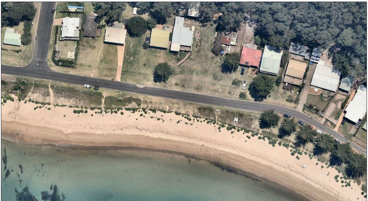
Image 7: Works area as of January 2020.
