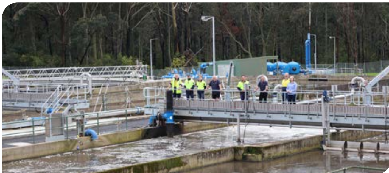
Image: It was a team effort to keep the Batemans Bay sewage upgrade flowing.
