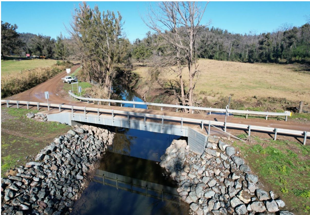
Photo A.7 – Reedy Creek bridge – a new concrete bridge is now in place and the approaches have since been sealed to reduce sediment loads into nearby waterways and better care for the new bridge
