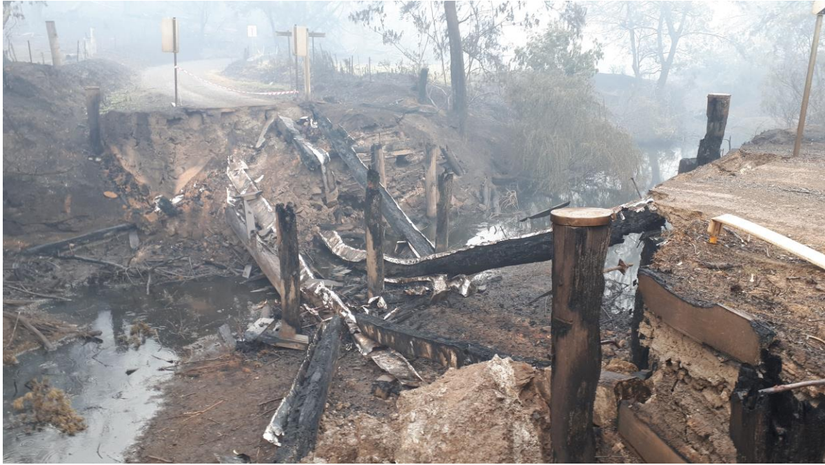
Photo A.6 – Reedy Creek bridge was completely destroyed during the bushfires requiring multiple temporary crossing structures to be built and rebuilt due to flooding damage prior to completion of the new concrete bridge
