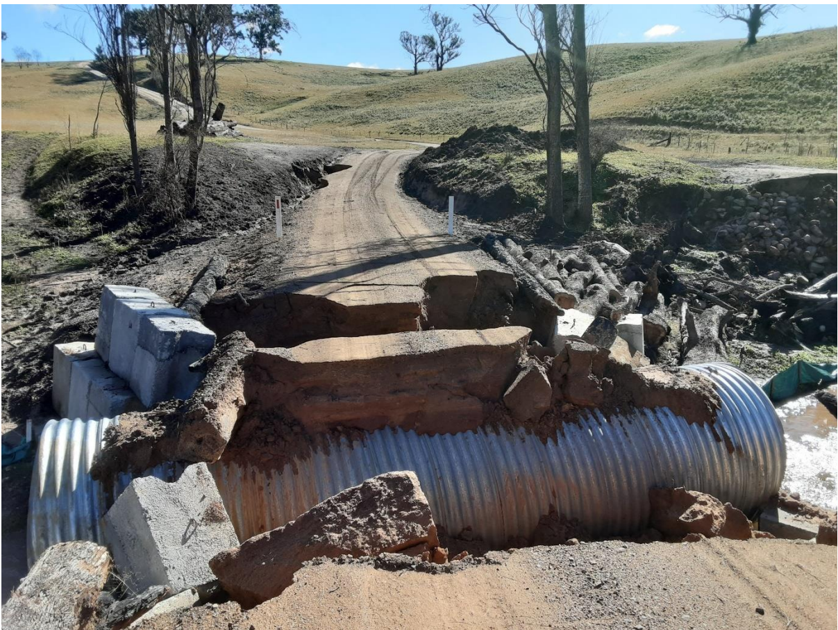
Photo A.30 – Belowra bridge Temporary access structures were repeatedly damaged by subsequent flood events
