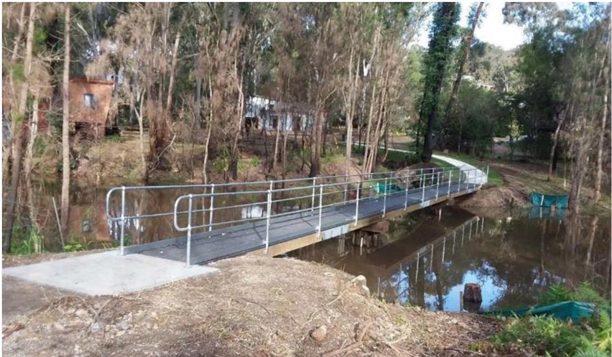
Photo A.3 Rosedale footbridge was replaced with a composite structure, in keeping with the surrounds, to reconnect the heavily impacted North and South Rosedale villages
