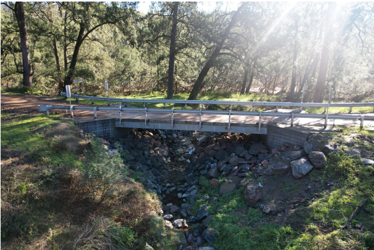
Photo A.9 – Peach Tree bridge – a new concrete bridge is now in place with sealed approaches
