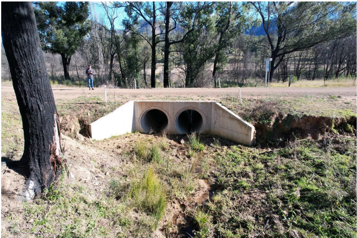
Photo A.28 – Four Gums bridge The bridge was replaced with a multiple cell concrete culvert
