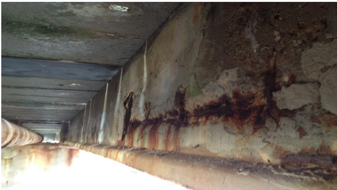
Candlagan Bridge Broulee – prior to replacement
