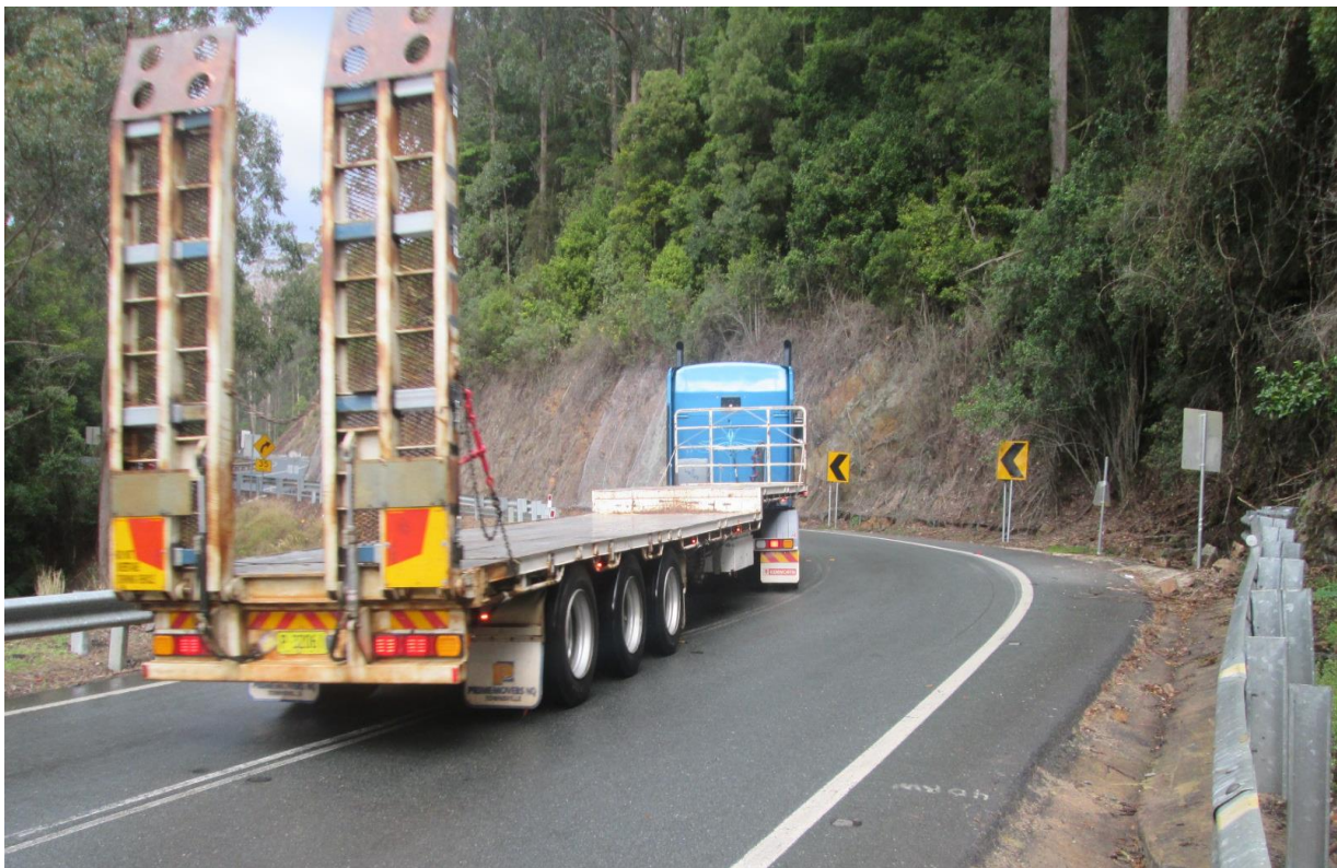
Normal semi-trailer crossing the centre-line on the Clyde Mountain to avoid hitting the guardrail at a high accident site – a short viaduct will provide a solution
