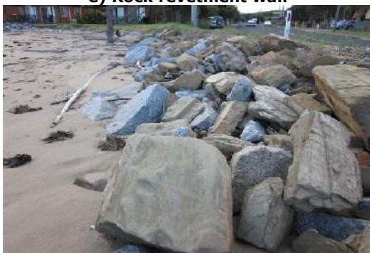
g) Rock wall armour properties are mixed
