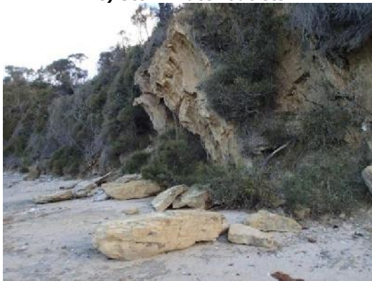
e) Backing rocky bluffs with rockfall
