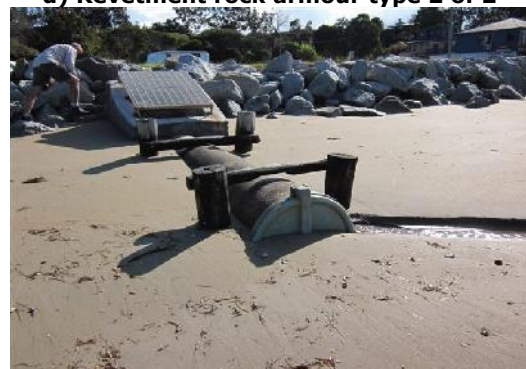
f) Stormwater outlet (blocked floodgate)
