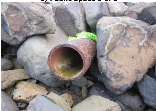
e) Typical local stormwater outlet
