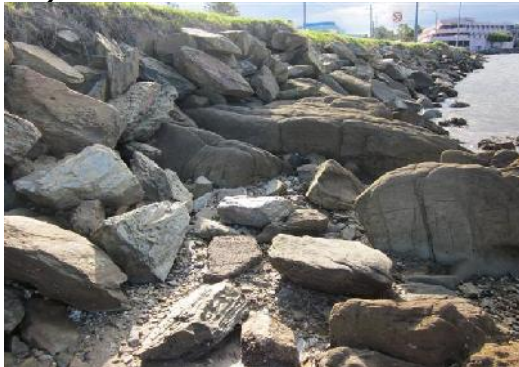
c) Revetment rock armour type 1 of 2
