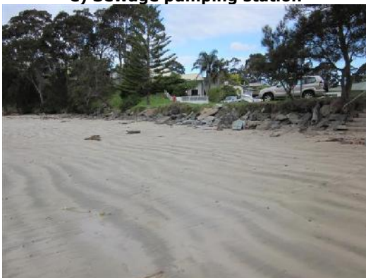
g) Southern end of rock revetment wall
