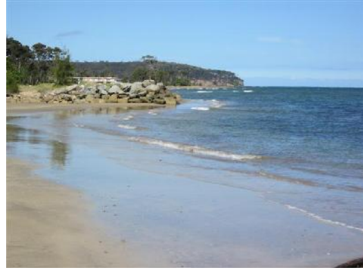
b) Unapproved groyne
