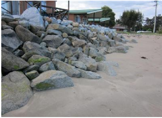
a) Eastern end of rock revetment wall
