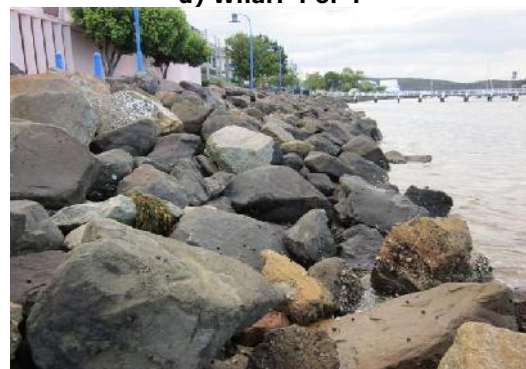
f) View of revetment wall looking north
