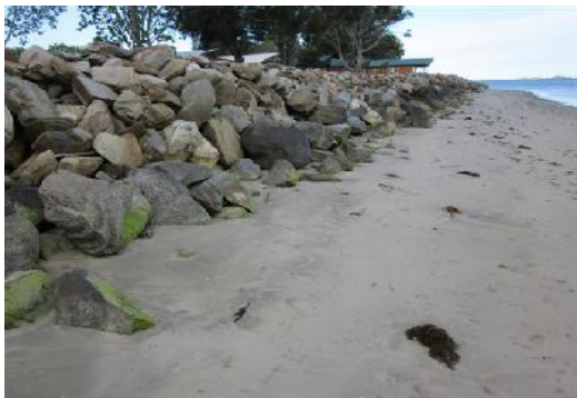
e) View of revetment wall looking east
