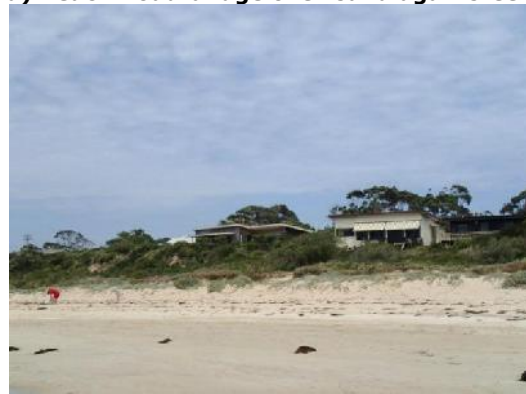
f) Houses at the northern end
