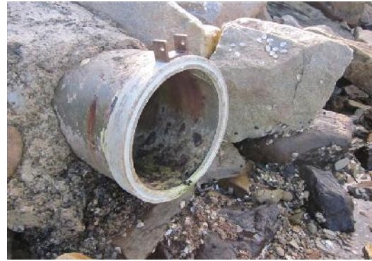
b) Stormwater outlet (missing floodgate)
