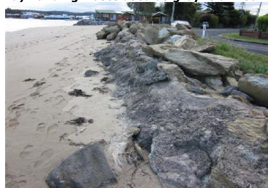
f) Wall armour is grouted together
