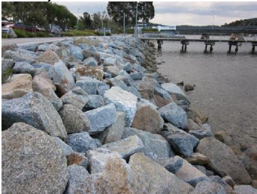
c) View of revetment wall looking west 1
