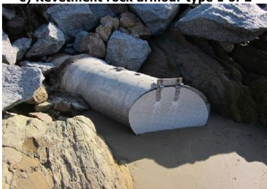
b) Stormwater outlet (blocked floodgate)
