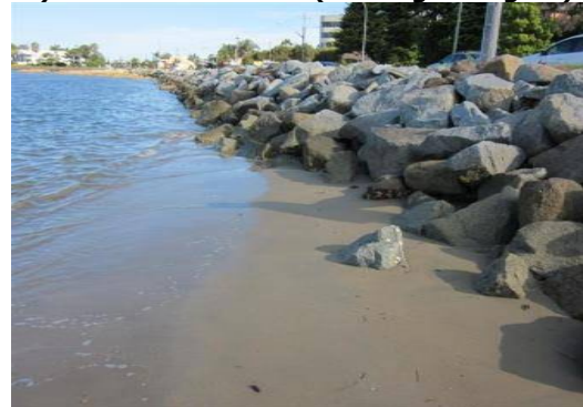
d) Revetment rock armour type 2 of 2
