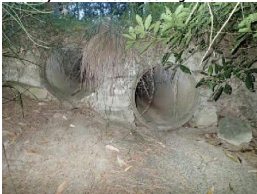
c) Stormwater outlets
