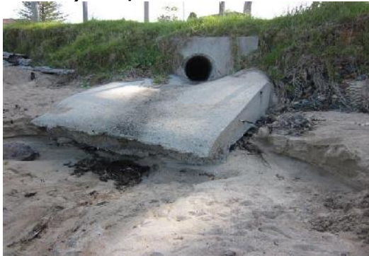
c) Stormwater outlet
