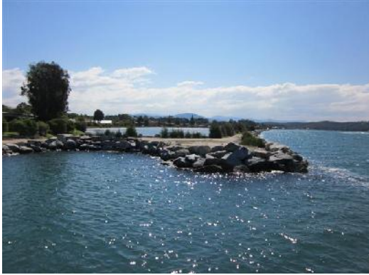
a) View of boat harbour looking west
