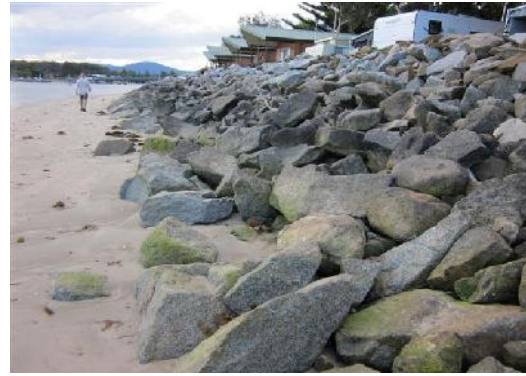
b) View of revetment wall looking west
