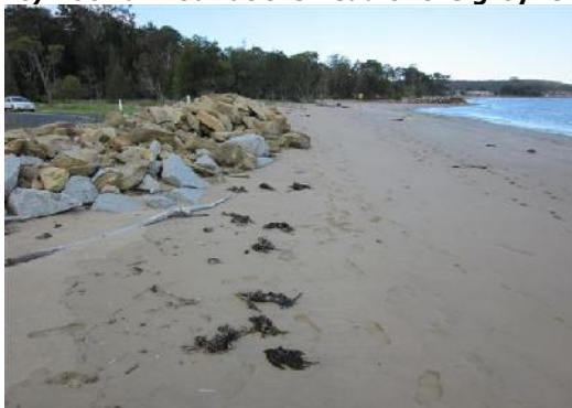
e) Rock revetment wall
