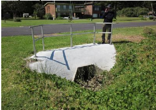
c) Stormwater Outlet 1
