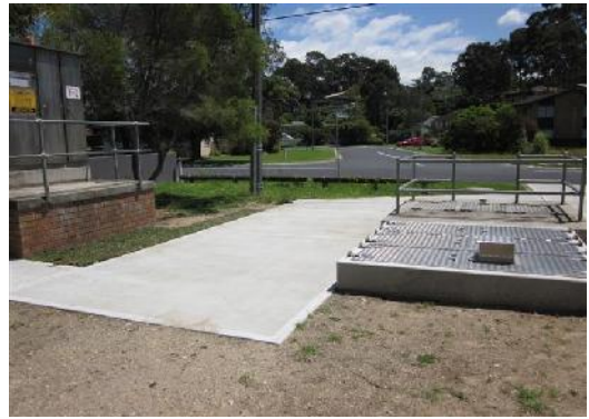
b) Sewage pumping station
