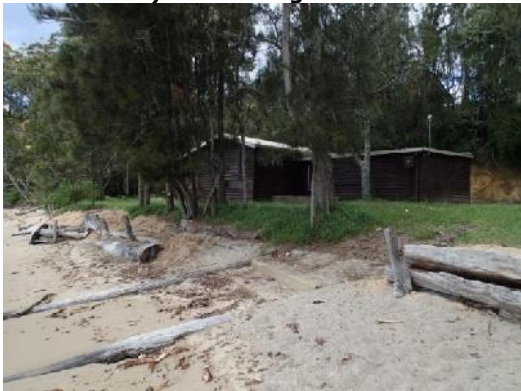
e) Wooden retaining wall at southern end
