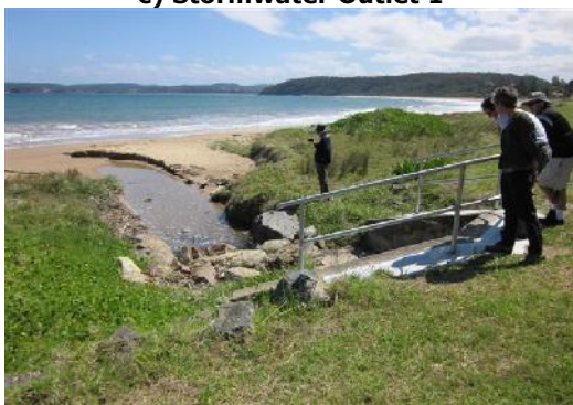
e) Stormwater Outlet 2
