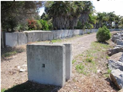
c) Concrete cube wall seaward of development
