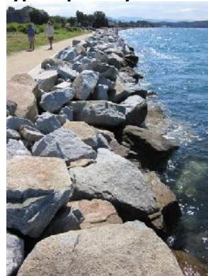
f) View of rock training wall looking west
