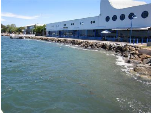
a) View of revetment wall looking south
