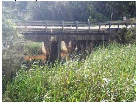
f) Box culverts under George Bass Drive
