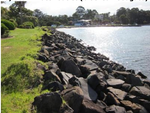
g) Eastern end of rock revetment wall
