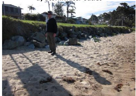
f) Northern end of rock revetment wall
