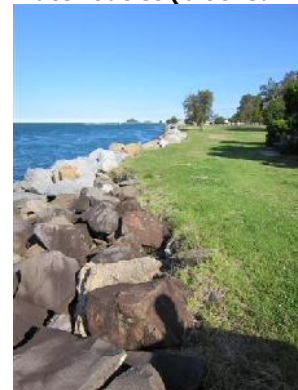
h) Western end of rock training wall
