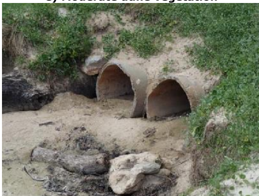
g) Stormwater outlets at the southern end
