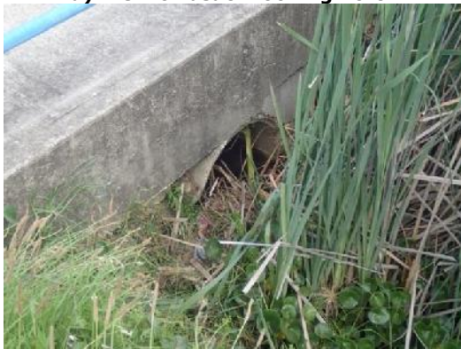
c) Blocked stormwater pit at southern end
