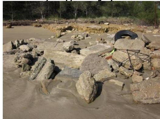
d) Building waste used as groyne armour
