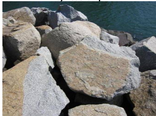
d) Typical primary rock armour
