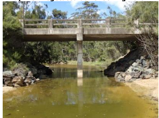
f) Durras Road bridge at southern end
