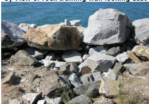
g) Typical secondary rock armour
