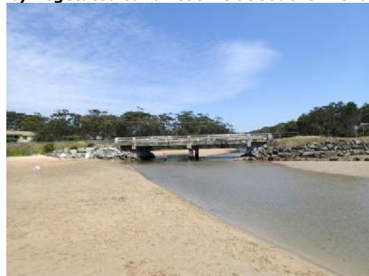
d) Beach Road bridge over Candlagan Creek
