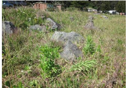
d) Partially buried rock revetment wall
