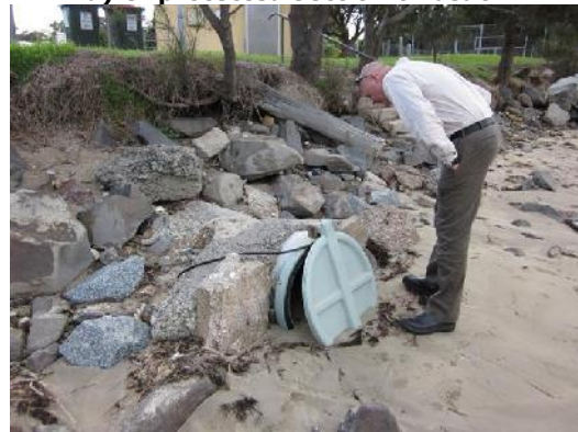
f) Stormwater outlet (blocked floodgate)
