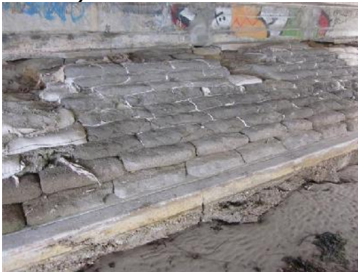
c) Scour protection at bridge abutments
