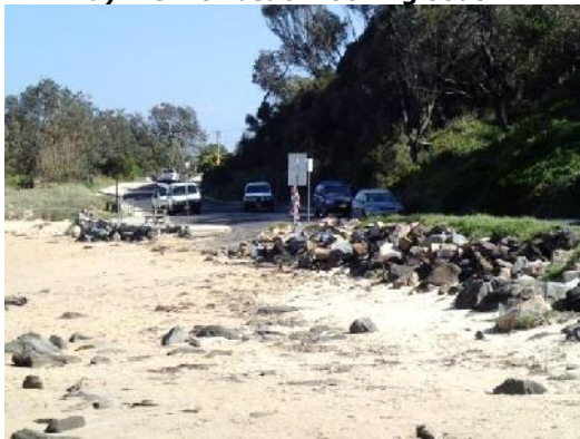
c) Boat ramp and rock revetment
