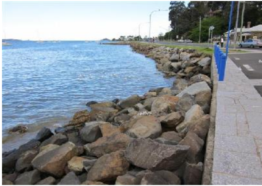
a) Western end of rock revetment wall
