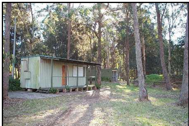
Batemans Bay BMX Track Amenities Building The maintenance responsibilities are shared between the Management Committee and Eurobodalla Shire Council.
